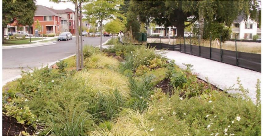
Figure 2. A completed natural drainage system
