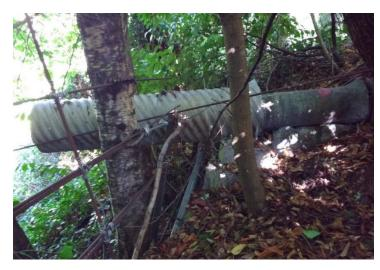
Water flows out the end of the pipe and drops onto the side of the canyon below. This causes significant erosion. SPU will "tightline" two drainage outfalls to prevent further erosion of the canyon while still delivering the water to the creek. Tightlines are essentially pipes placed on the ground surface that connect to a pipe exiting from underground such as an outfall.
