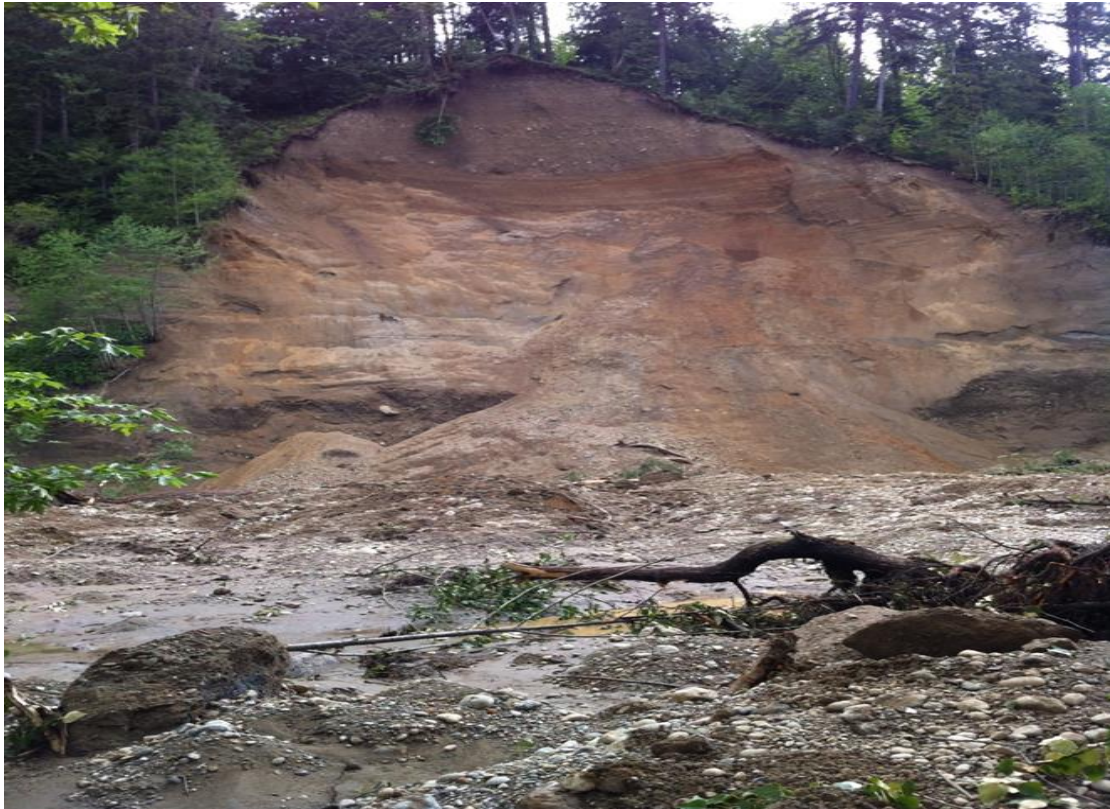
Figure 4. Photograph of Landslide that covered and/or moved all 13 accelerometers in site C.
