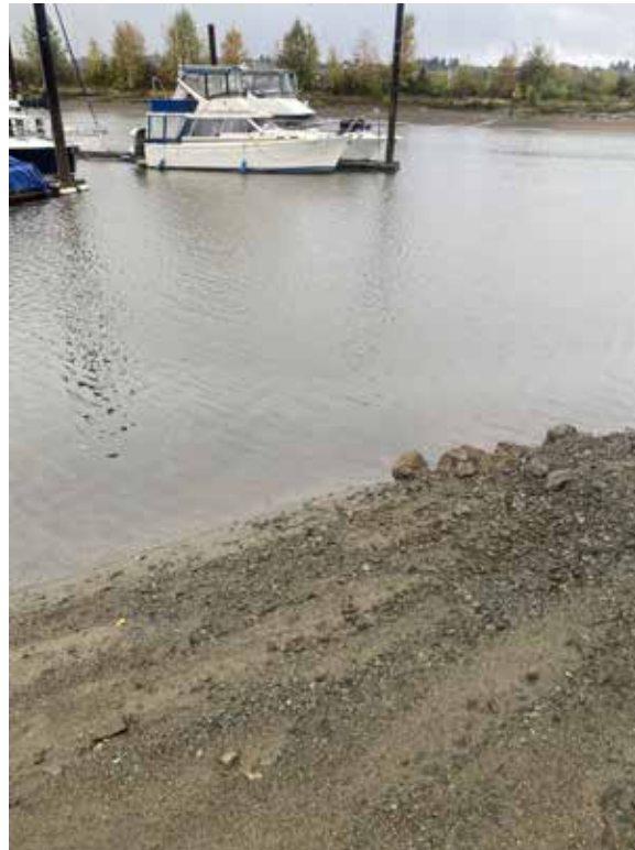
Photo Location 3. Northeast shoreline of Restored Shoreline and Intertidal Area, looking east
