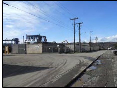
Figure 2: S Garden St Metals Storage
