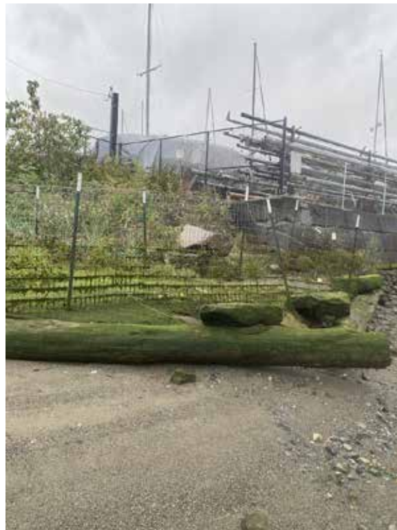
Photo Location 1. Northeast shoreline of Restored Shoreline and Intertidal Area, near South Park Marina
