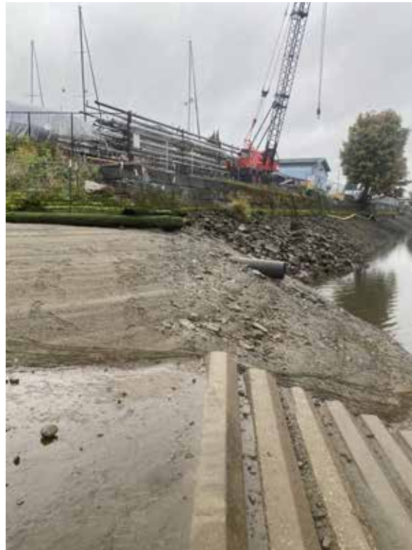
Photo Location 3. Northeast shoreline of Restored Shoreline and Intertidal Area, looking north
