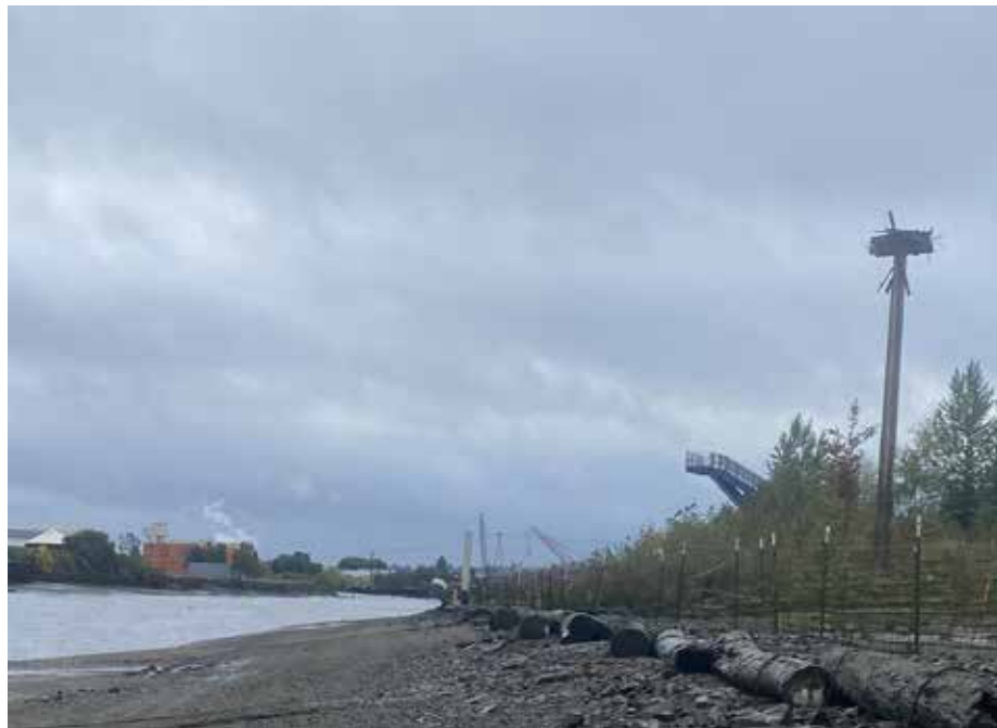
Photo Location 4. North end of DU1 cap, looking south
