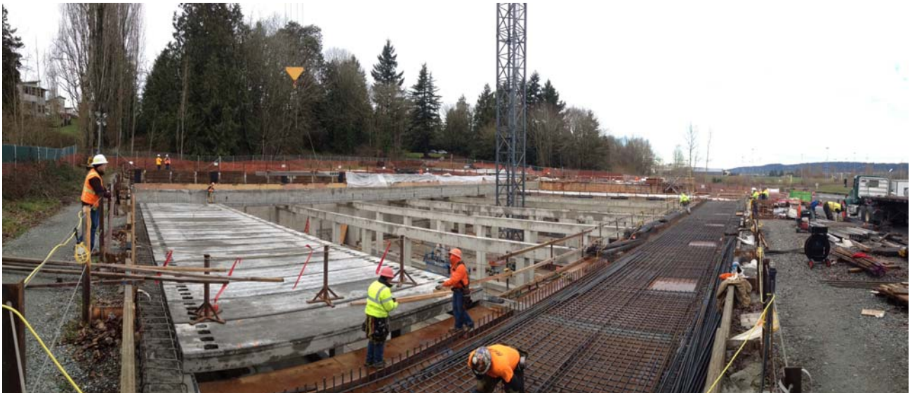
Figure 4-8. Windermere CSO Reduction Project Construction, February 2014
