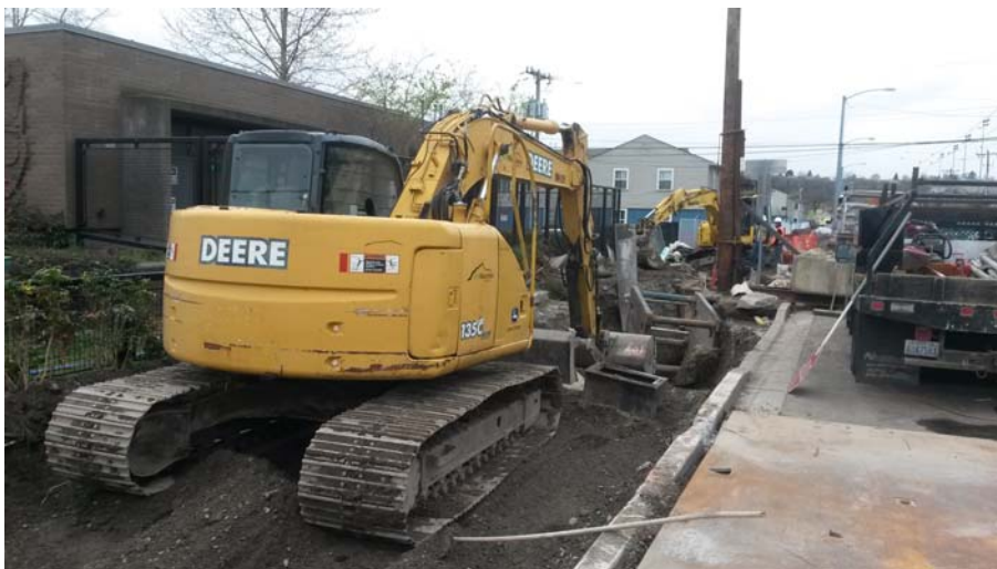
Figure 4-11. 52 nd Ave S Conveyance Project Construction, March 2014
