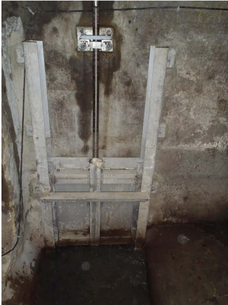
Figure 4-1. New Slide Gate in Basin 13 (Windermere Area)
