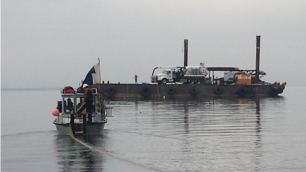
Figure 4-15. Outfall 95 Rehabilitation Project
