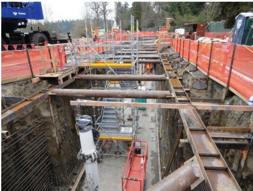
Figure 4-10. Genesee (CSO 9A) CSO Reduction Project Construction, February 2014
