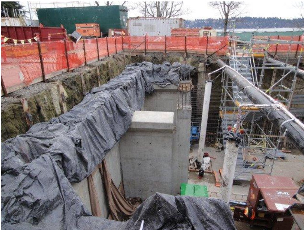
Figure 4-9. Genesee (CSO 11A) CSO Reduction Project Construction, February 2014
