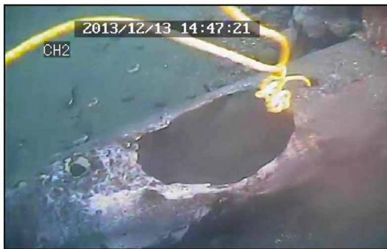
Photo 4: Clean interior & exterior repair area prior to sleeve installation.
