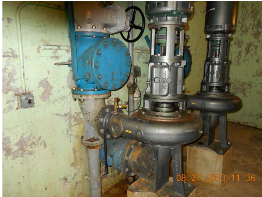
Figure 4-12. Pump Station 9 Rehabilitation Project
