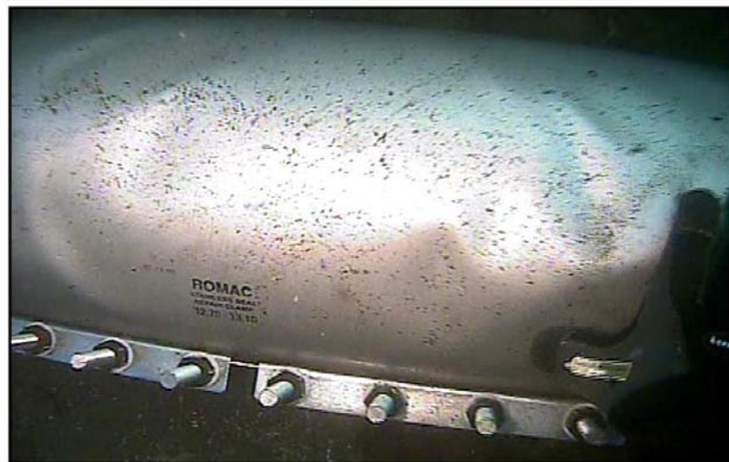
Photo 5: ROMAC repair sleeve installed.
