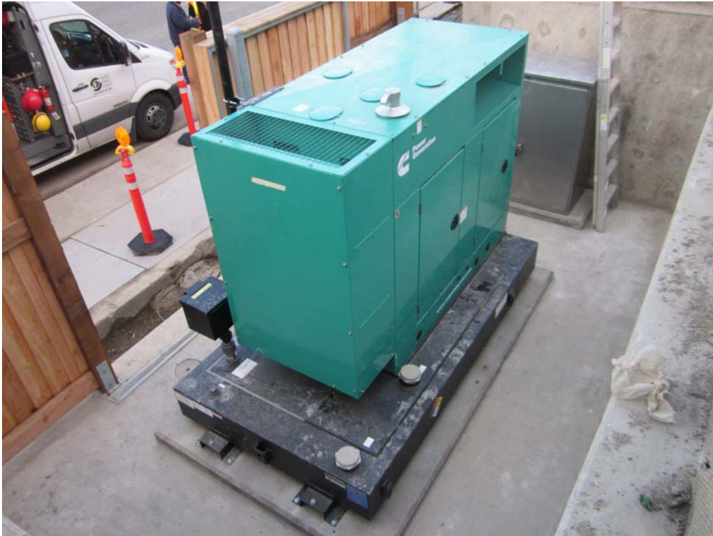
Figure 4-13. Pump Station 39 Backup Generator
