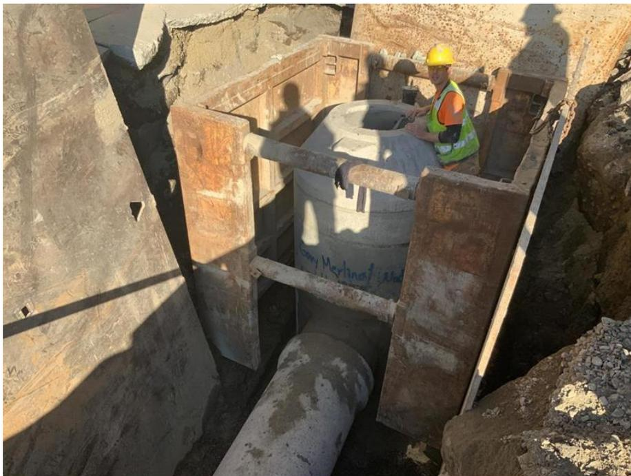
Figure 4-6. Central Waterfront Construction – Maintenance Hole Installation
