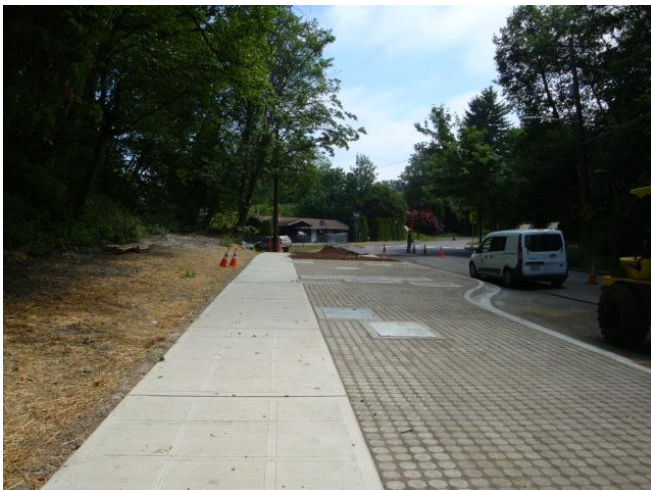
Figure 4-3. New Delridge Diversion Structure (upper) and Finished Appearance (lower)
