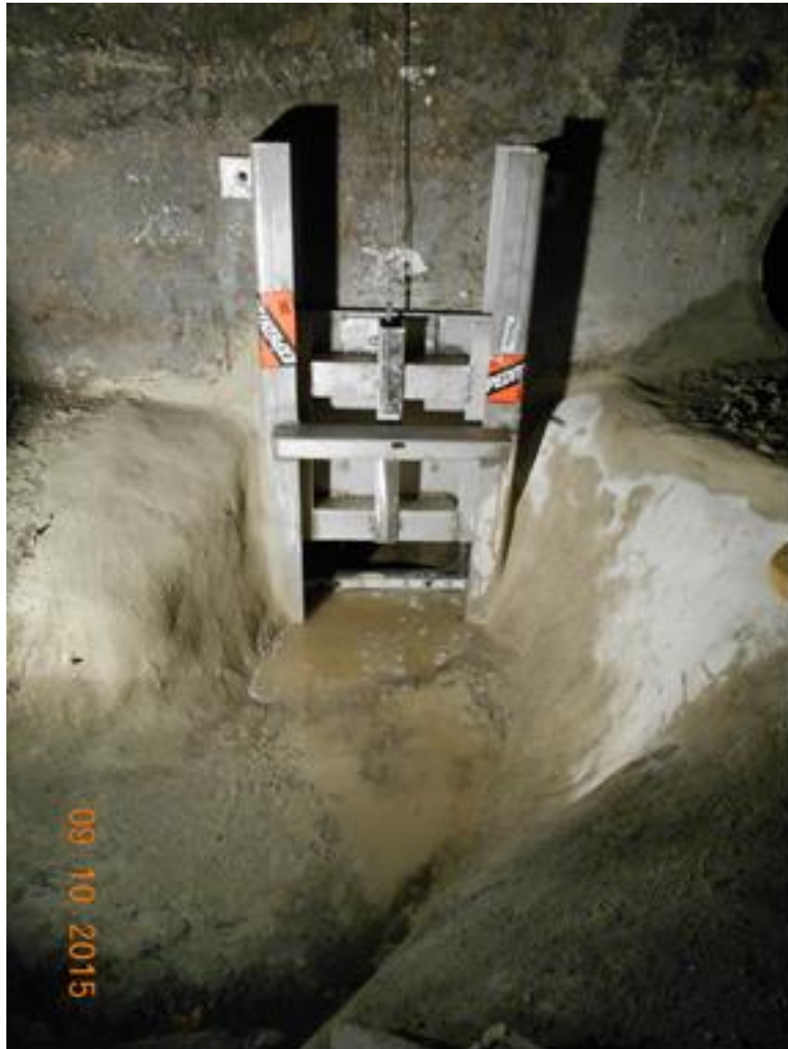
Figure 4-2. New North Union Bay Automated Gate
