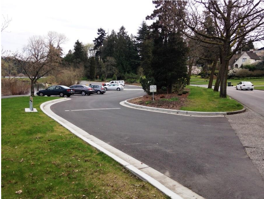
Figure 4-10. Completed Genesee CSO Storage Facility 9A
