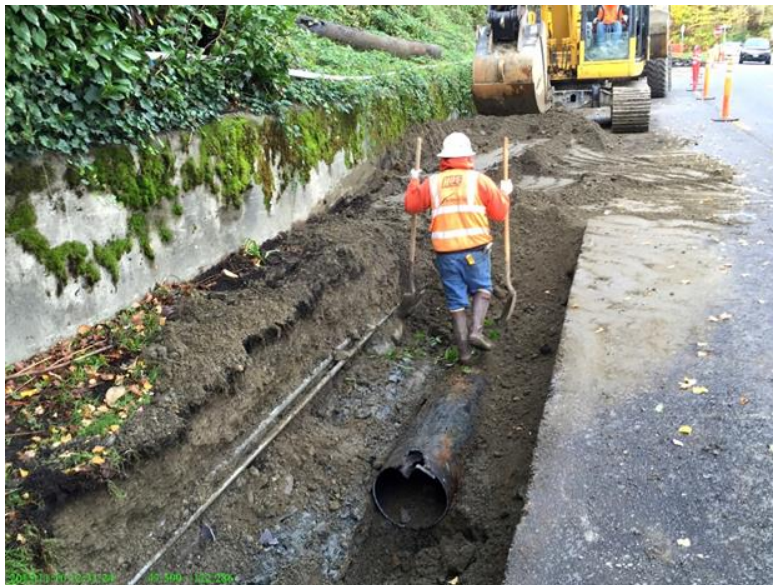
Figure 4-4. Combined Sewer Replacement in Leschi
