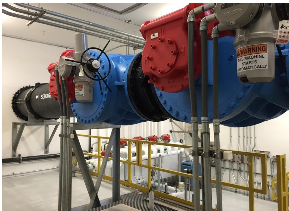
Figure 4-9. Completed Windermere Facility Vault – Mechanical Room
