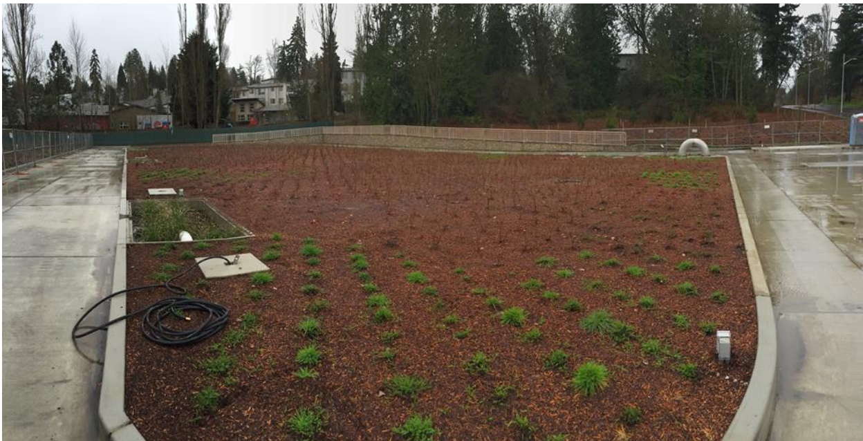
Figure 4-8. Completed Windermere CSO Storage Facility
