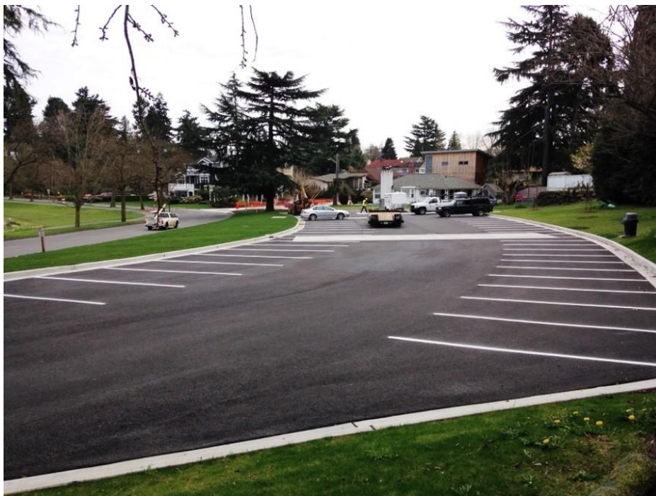
Figure 4-11. Completed Genesee CSO Storage Facility 11A
