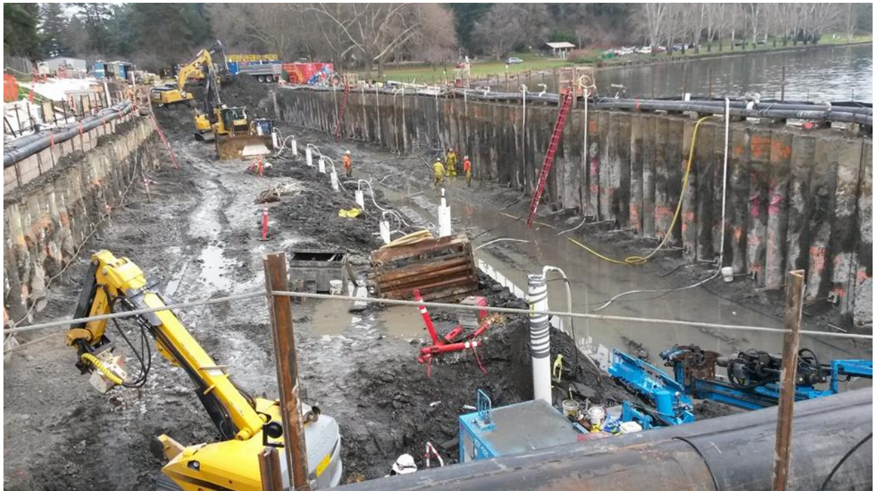
Figure 4-12. North Henderson CSO Storage Facility during Construction
