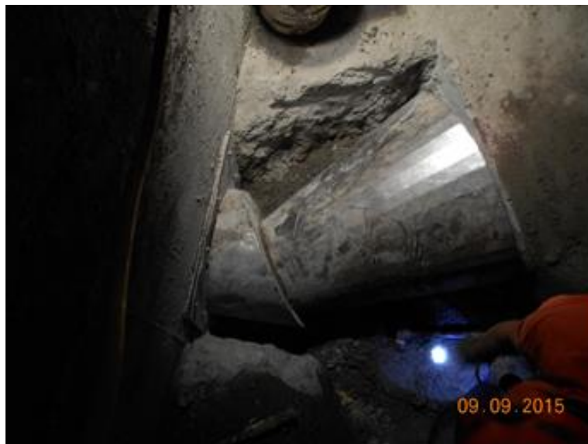
Figure 4-1. Former North Union Bay HydroBrake
