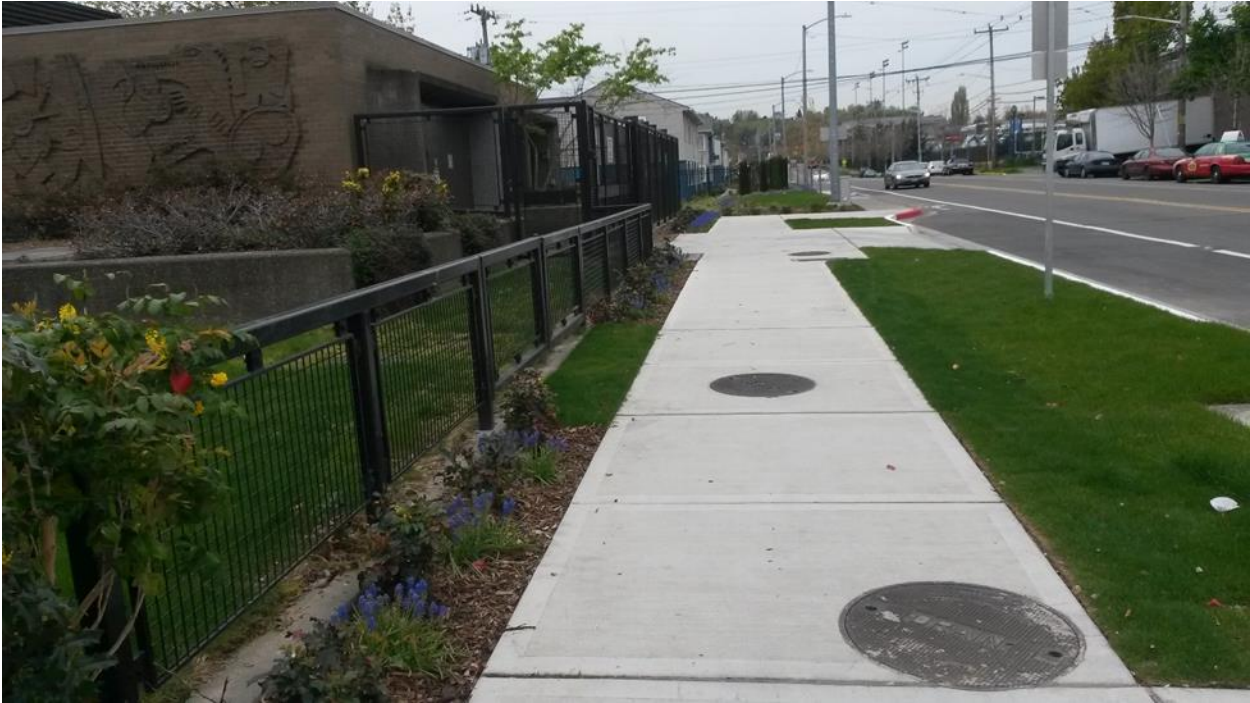
Figure 4-14. Completed 52 nd Ave S Combined Sewage Conveyance Project
