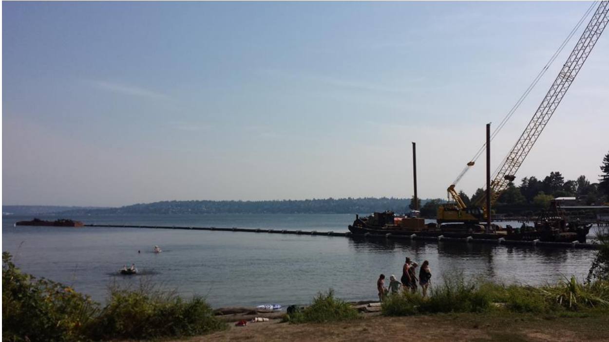
Figure 4-13. CSO Outfall 44 during Construction
