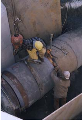
Installation of the Tolt Transmission Pipeline
