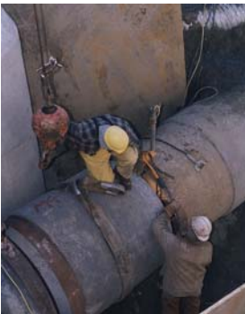
Installation of the Tolt Transmission Pipeline
