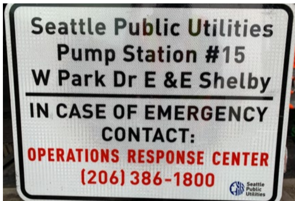
Figure 11-4 Typical Pump Station Identification Signage
