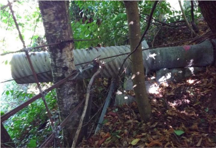
Water flows out the end of the pipe and drops onto the side of the canyon below. This causes significant erosion. SPU will “tightline” two drainage outfalls to prevent further erosion of the canyon while still delivering the water to the creek. Tightlines are essentially pipes placed on the ground surface that connect to a pipe exiting from underground such as an outfall.
