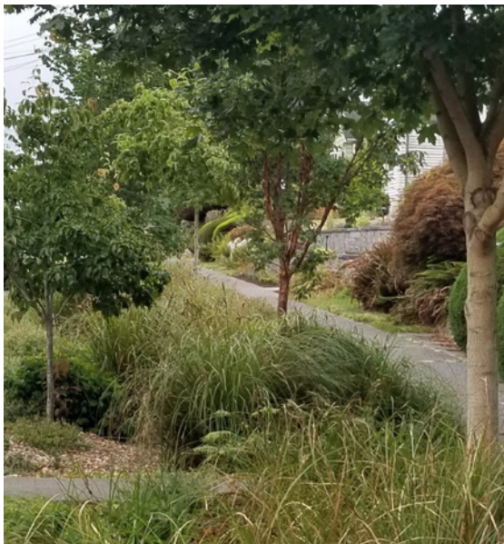
A completed natural drainage system on a residential street.
