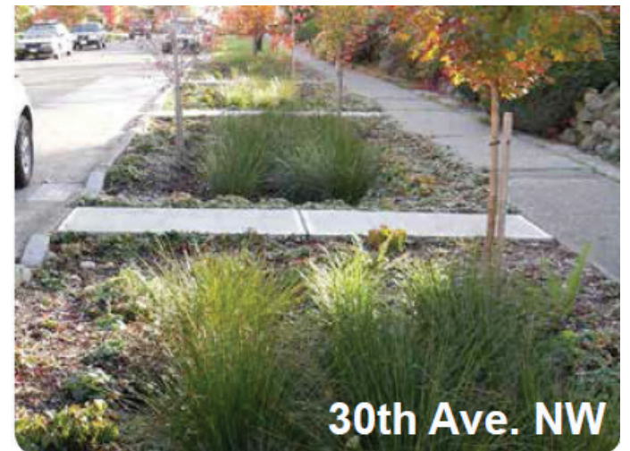
These images show examples of NDS in Seattle. NDS in your neighborhood may look different. (Credit: Seattle Public Utilities)
