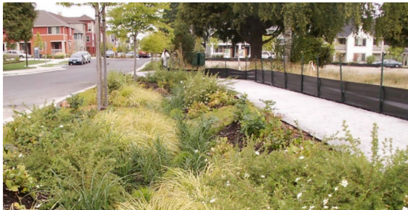
A completed natural drainage system.
