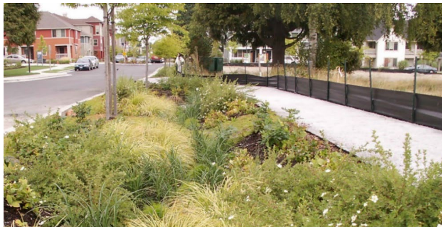
A completed natural drainage system.
