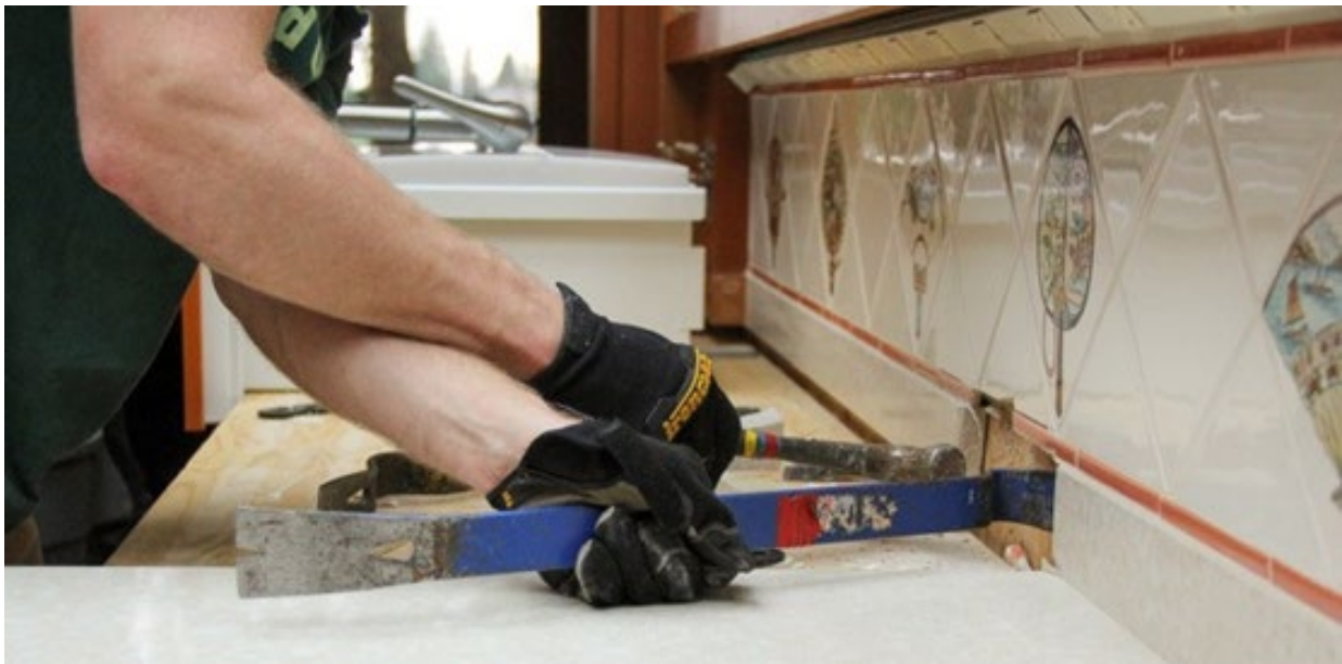
Kitchen tile removal for salvaging (Source: Second Use, 2020)
