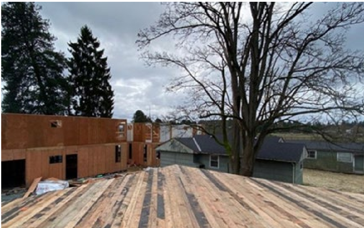
Construction site for three new homes using reclaimed lumber in West Seattle (Source: Seattle Sledge, 2019)
