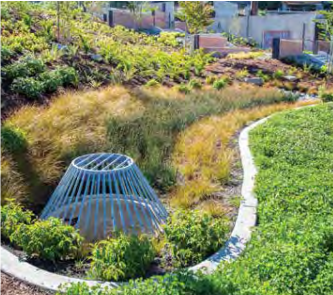
The Murray Pump Station in West Seattle features a green roof, permeable pavement, a bioswale, and two tree box filters that collectively manage runoff from a half acre adjacent to the facility.
