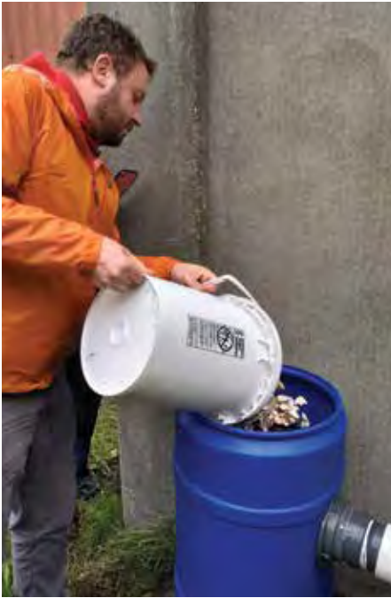
Workshop volunteer adds oyster shells to remove heavy metals from stormwater.
