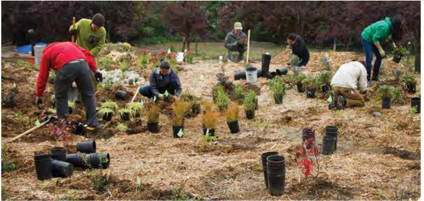
Volunteers and partners help install a 2,200 square foot rain garden, named “Reclaiming Home,” by local students who worked on the design.
