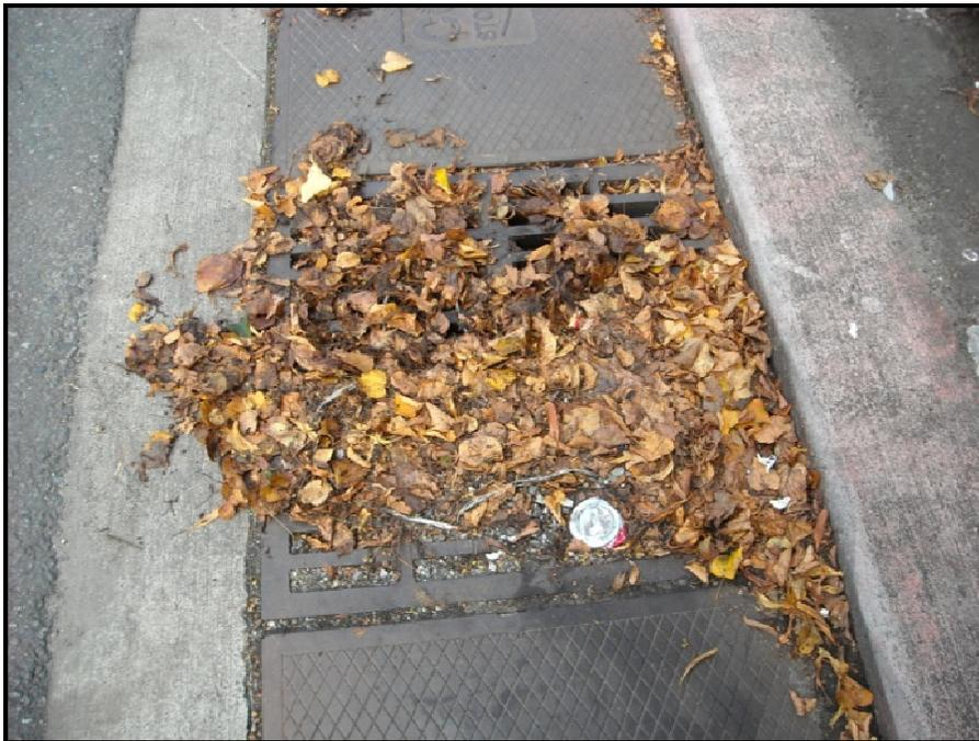
Figure 5.3.3b. Inlet grate clogging at CBSF1 during mid-winter conditions
