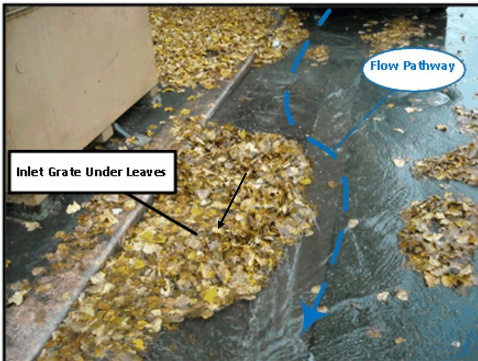
Figure 5.3.3d. Partial inlet grate blockage at CBSF2 showing flow bypassing inlet
