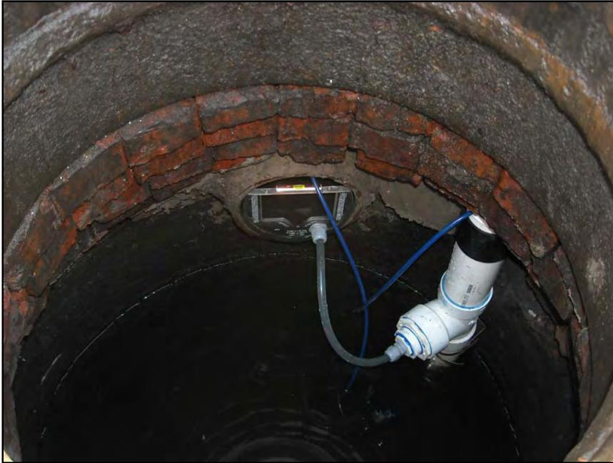
Figure 2.3.1b. Photo of Bypass Weir in CBSF2
