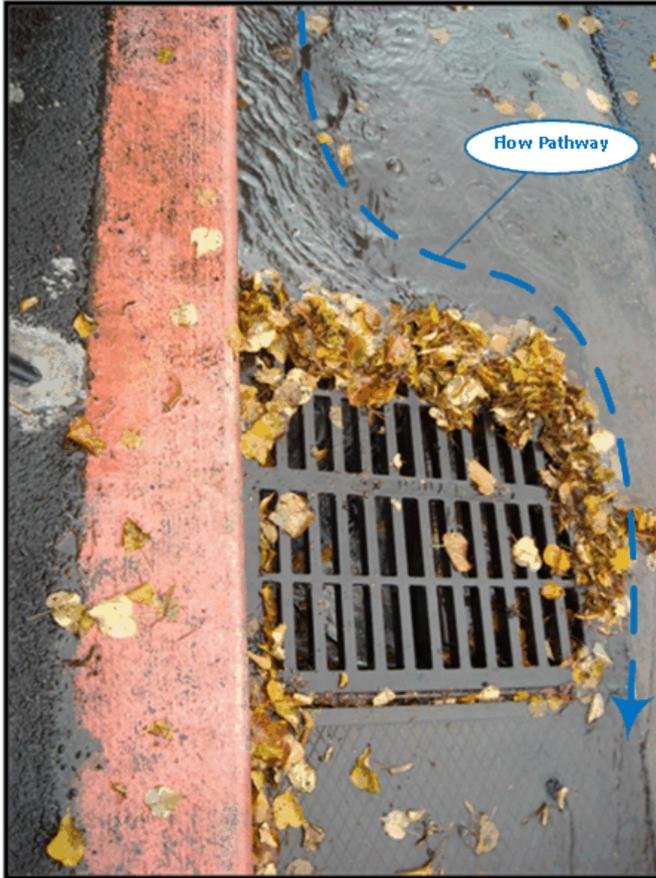
Excessive inlet grate blockage is attributed to three factors of the inlet grate design of the monitored units:
