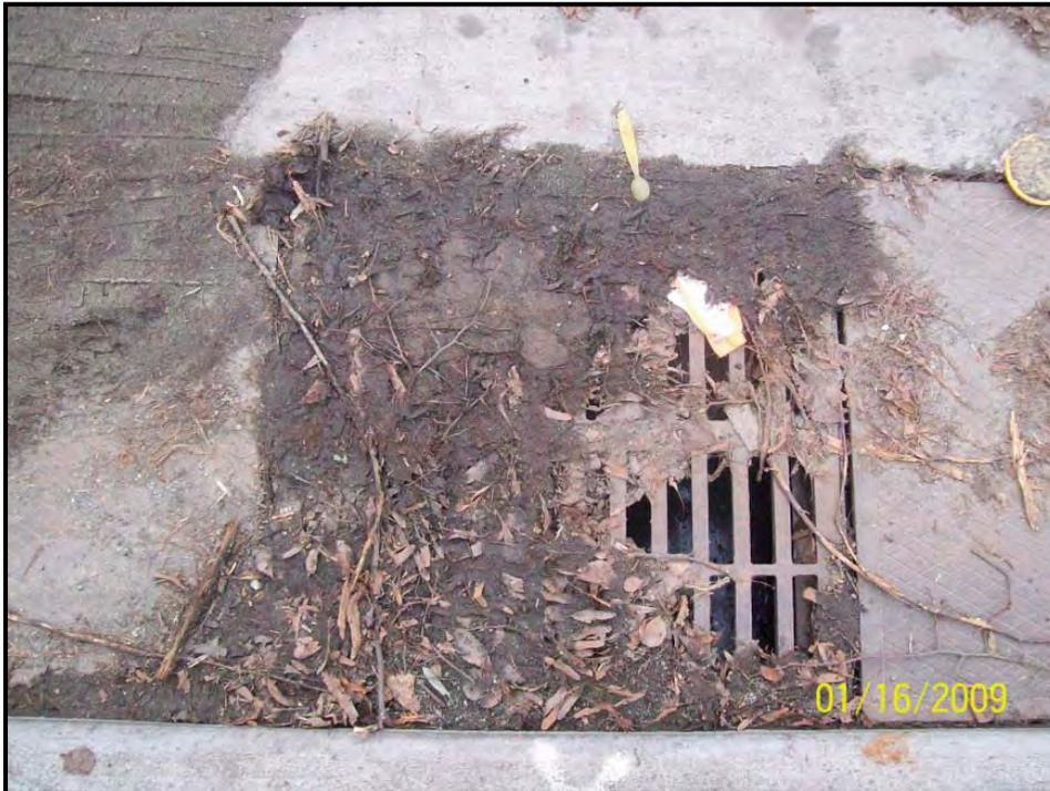
Figure 5.3.3c. Complete inlet grate clogging at CBSF2 showing flow bypassing inlet
