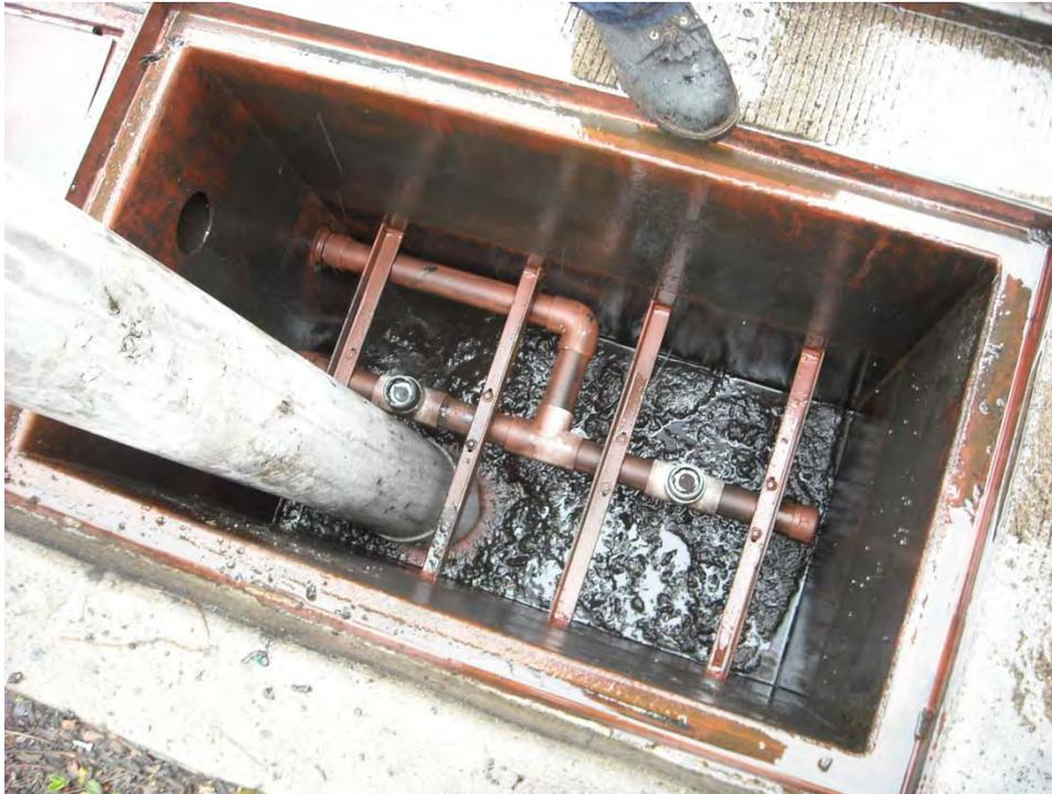
Maintenance was performed annually, or sooner, although the one observable sediment loading trigger for maintenance provided by the manufacturer [ $>0.25$  inches sediment accumulation on top of the cartridge (Darcy, 2012)] was not exceeded.
