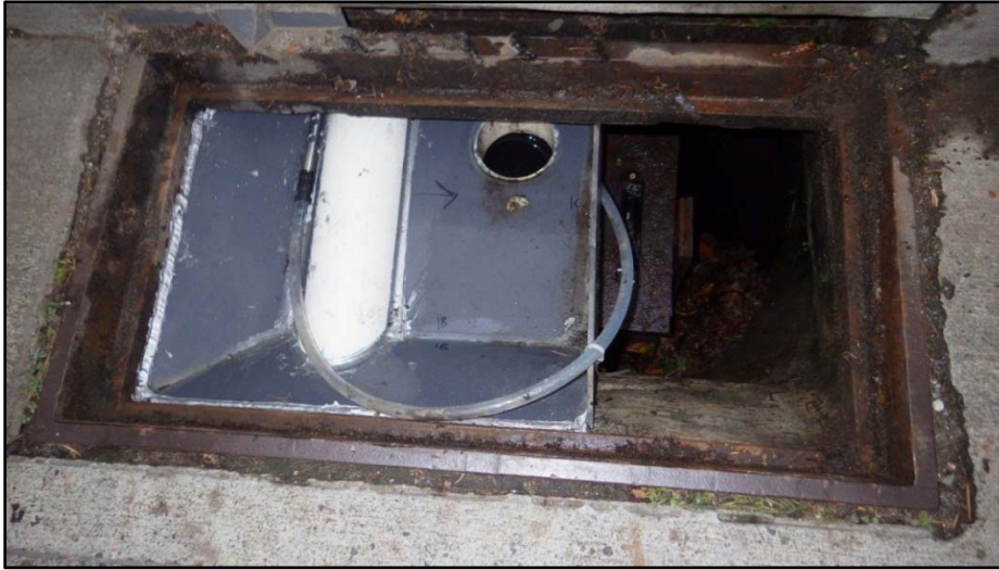
Figure 8. Sampling tray installed in inlet (inlet grate removed).
