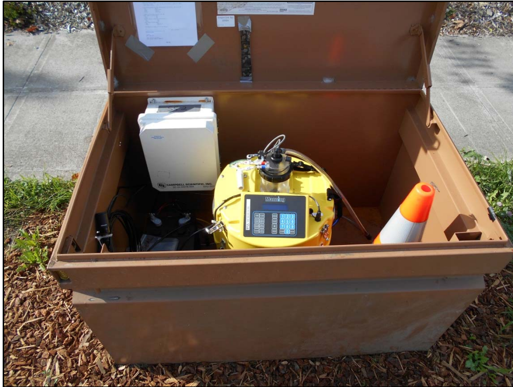
Figure 10. Cabinet containing sampler (yellow) and data logger enclosure (white).
