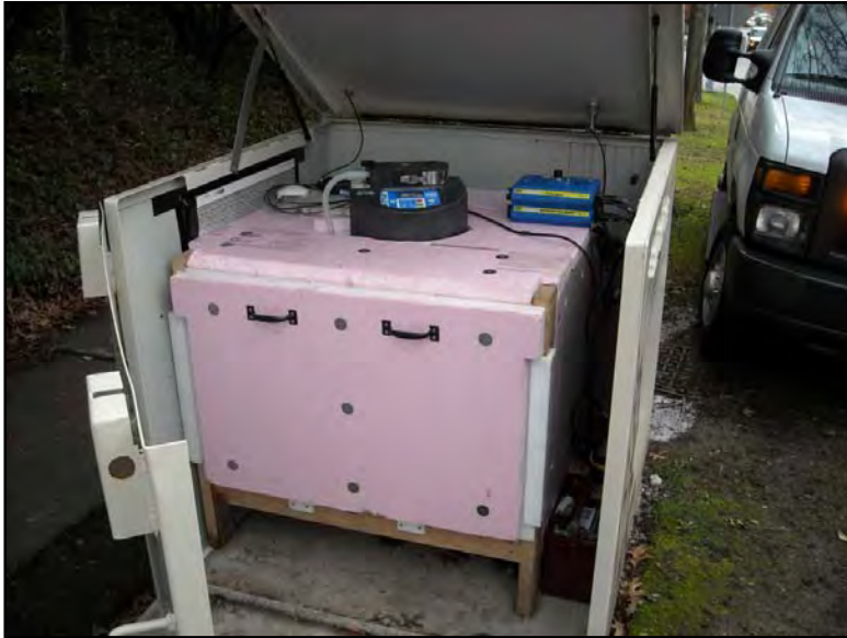
Figure 2.2.2.b. Photograph of C1 Equipment Cabinet
