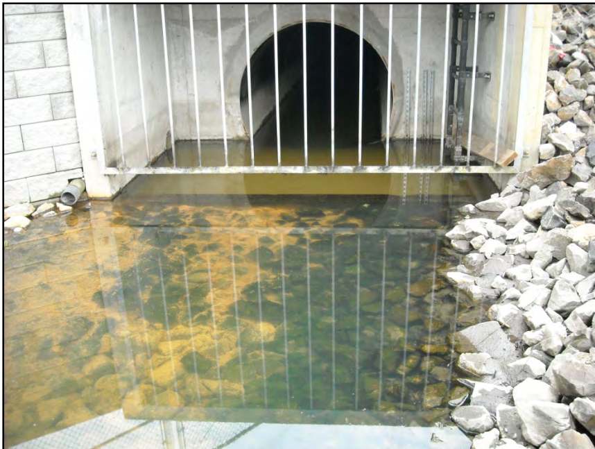
Figure 2.2.2.3c. Photograph of I1 Diversion Structure and Outfall
