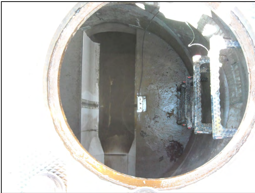
Figure 2.2.2.1b. Photo of R1 Palmer-Bowlus Flume
