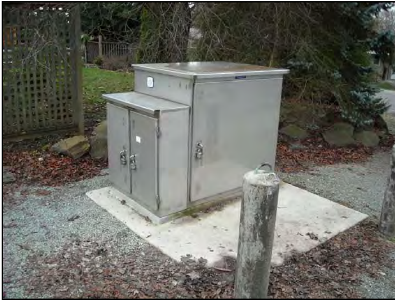
Figure 2.2.2.1c. Photo of R1 Equipment Cabinet
