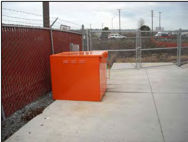
Figure 2.2.2.3d. Photograph of I1 Equipment Cabinet
