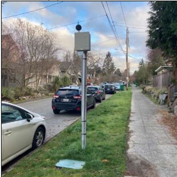
Photo 1. Equipment at Location 1
