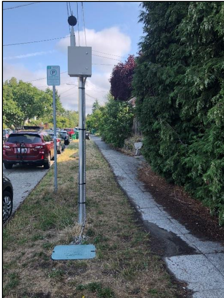
Photo 1. Equipment at Location 1
