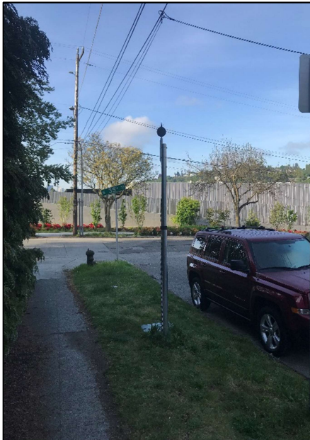
Photo 1. Equipment at Location 1
