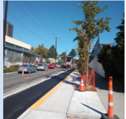
Before and After: Bus bulb - Northbound 12th Ave and NE 66th St
