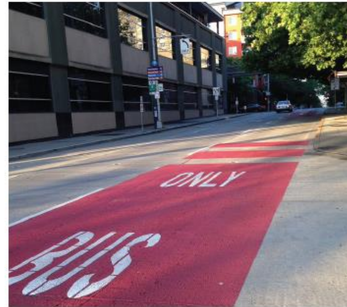
Red bus-only lane paint
