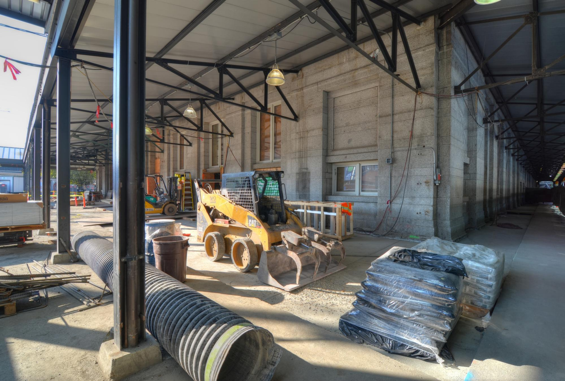
The new ring beam and slab on grade wraps around the east side of the building.
