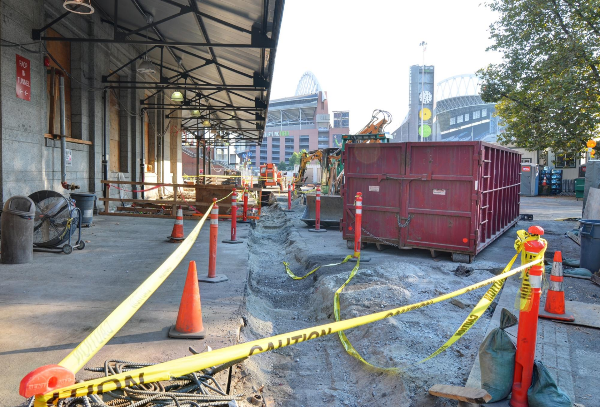
Some of the new upgrades along the west side of the station include installation of geothermal wells, gas and plumbing lines, seismic ring beams, reinforced ground slabs and utility vaults.
