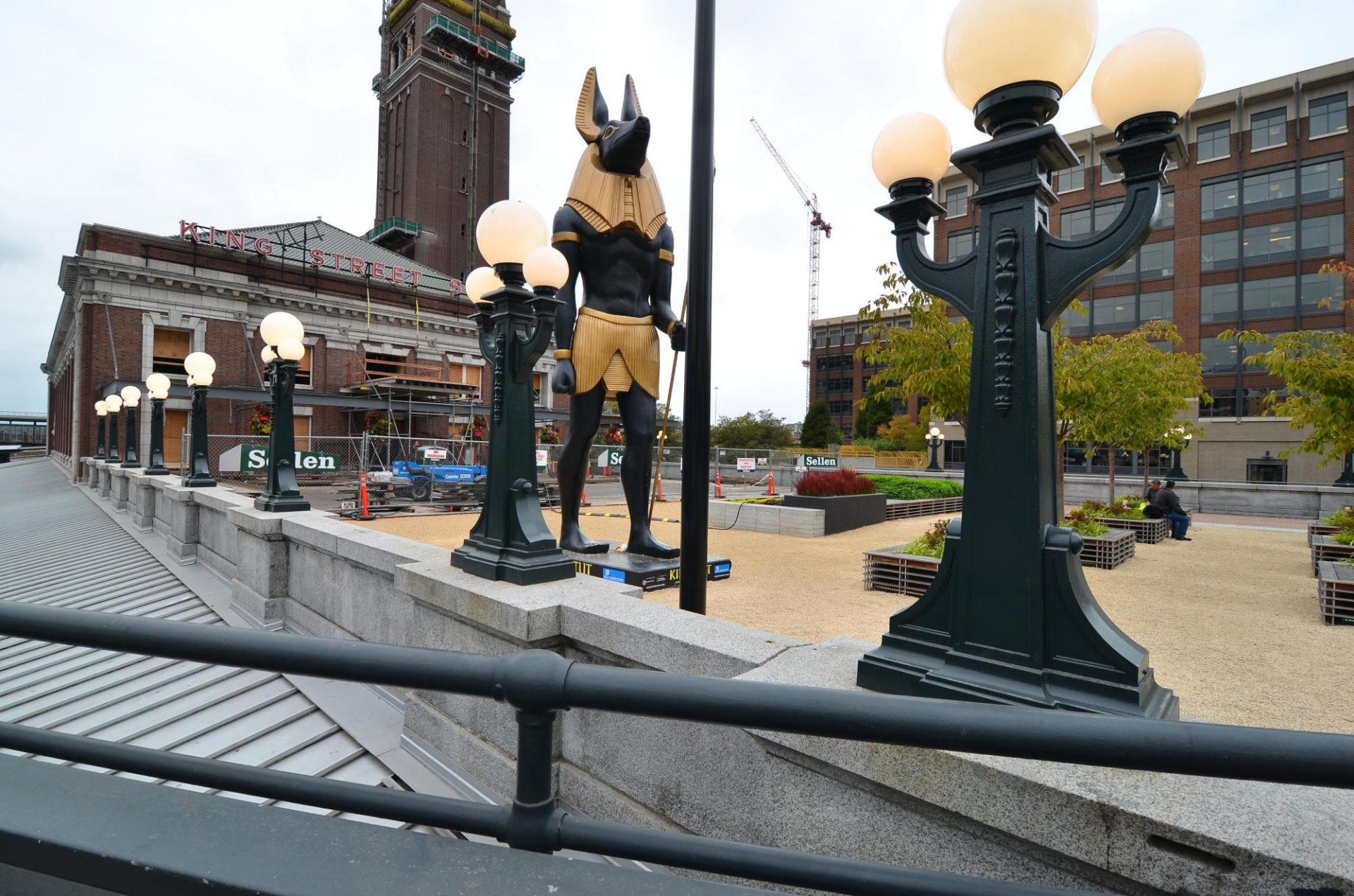
Balustrade light posts are lit with efficient LED modules. Both sides of the granite balustrade have been cleaned with approved chemicals by the Pioneer Square Preservation Board.
