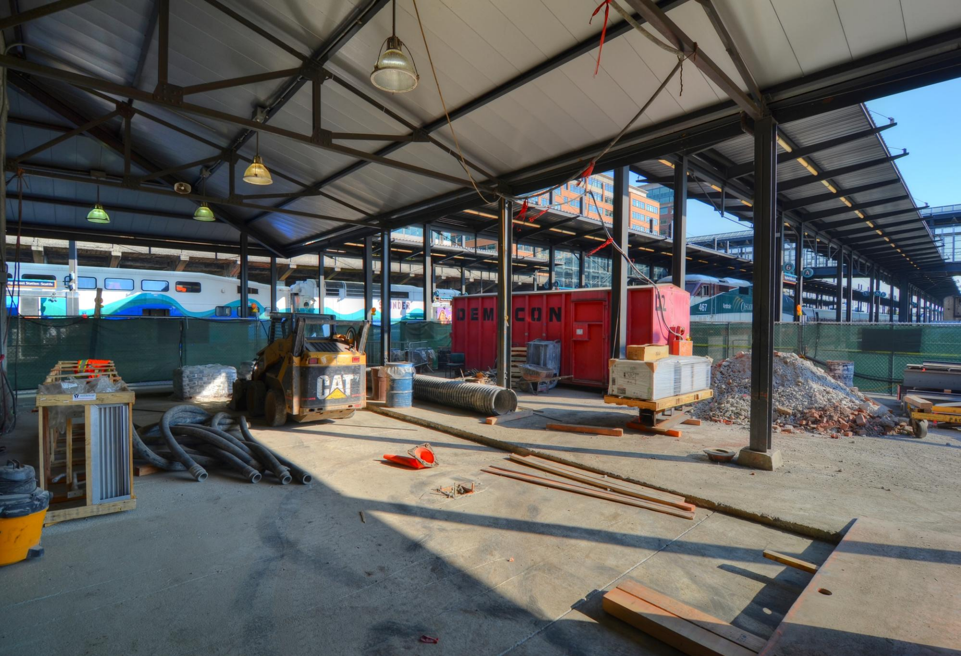
New lighting will be installed beneath the canopy. The ring beam and reinforced slab on grade were recently installed.
