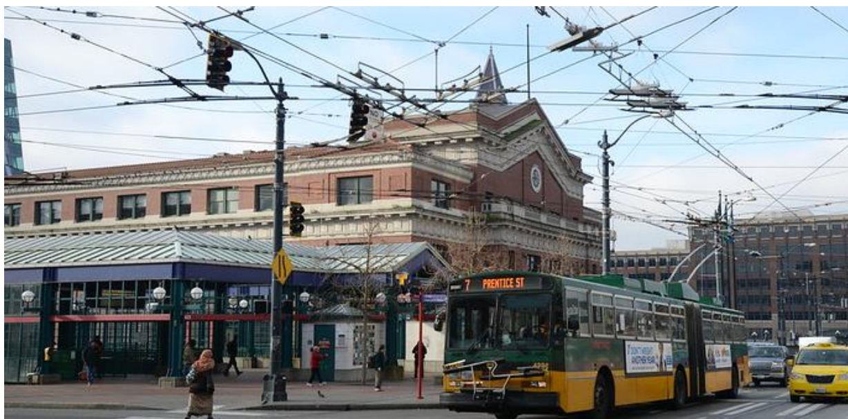
Union Station in the International District
