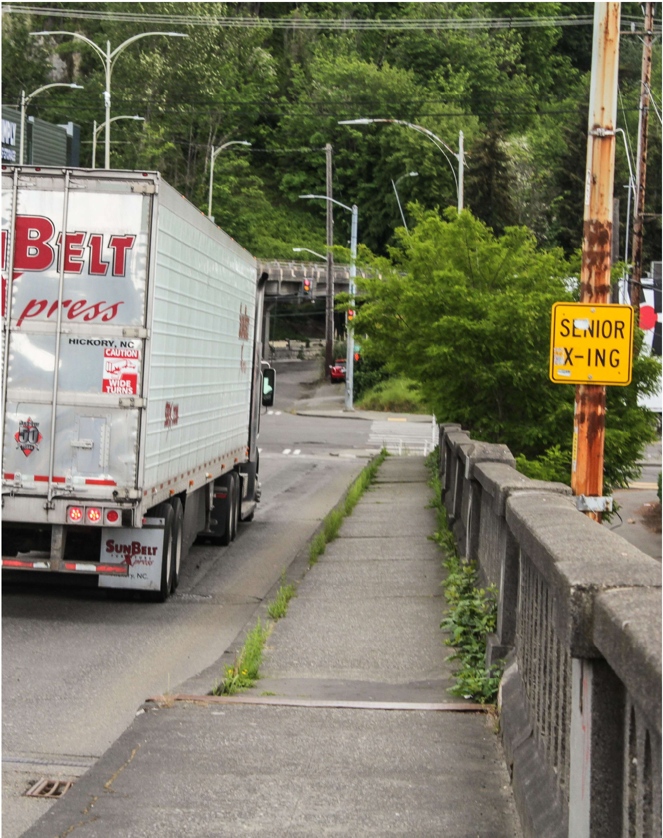
A truck crosses the Magnolia Bridge
