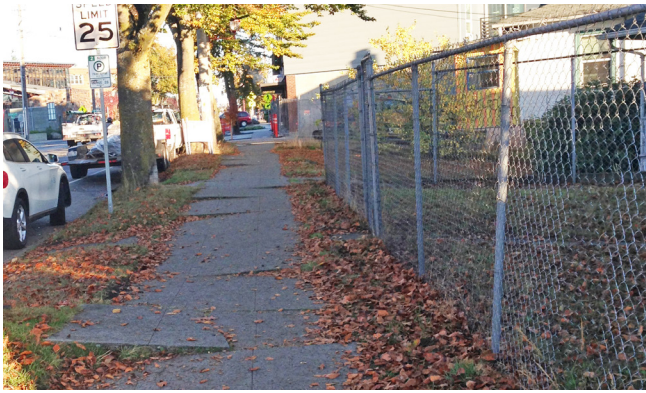
Sidewalk uplift, a trip hazard for all, can create a complete barrier to people who use mobility devices.
