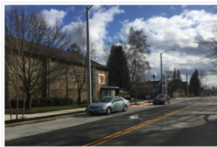
Complete three-lane roadway near 23rd Ave and E Olive St
