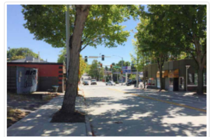
Completed 23rd Ave and E Cherry St intersection
