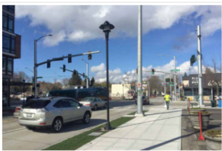
Completed 23rd Ave and E Union St intersection
