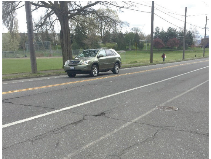
Swift Ave S / S Myrtle St / S Othello St needs to be repaved
