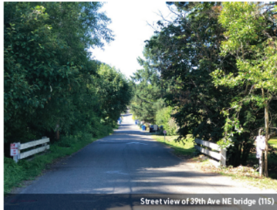
Street view of 39th Ave NE bridge (115)
