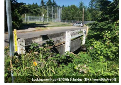
Looking north at NE 105th St bridge (104) from 40th Ave NE
