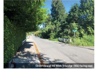
Street view of NE 105th St bridge (104) facing east
