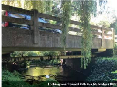
Looking west toward 45th Ave NE bridge (109)
