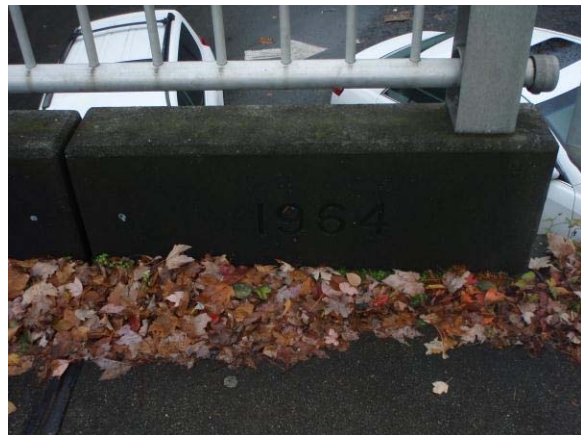
Photo 4. Detail of date inscription (1964) on south end of sidewalk (east side); this sidewalk handrail style is part of the 1963 design and is based on Standard Bridge Railing Type 3-A.
