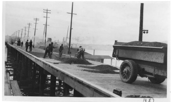
Photo 6. Note the original timber trestle supports and the gap between the West and East Bridges (Seattle Municipal Archives Photograph No. 57503). View to the south showing paving of the original West Bridge in 1924. 1924
