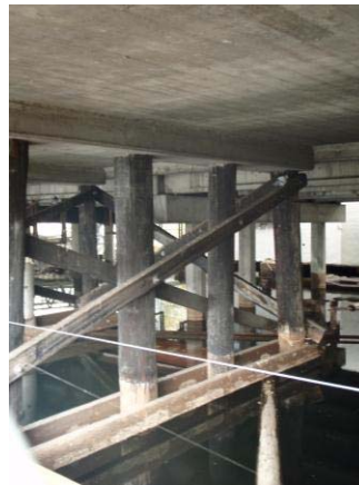
Photo 4. Note the timber pilings and cross-bracing; concrete piling bents for the East Bridge are visible in the background. View to the east showing a typical bent of the West Bridge. 2011
