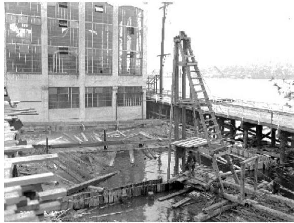
Photo 6. This shows the pilings and cross-beam supports for the original East Bridge (Seattle Municipal Archives Photograph No. 1364).
