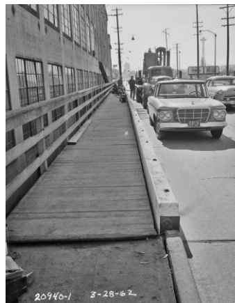
Photo 8. The wooden handrail and traffic curb date to the earlier (c.1917) bridge at this location. This handrail was replaced in 1963 except at the approaches. The traffic curb was replaced in 1988 (Seattle Municipal Archives Photograph No. 70916).
