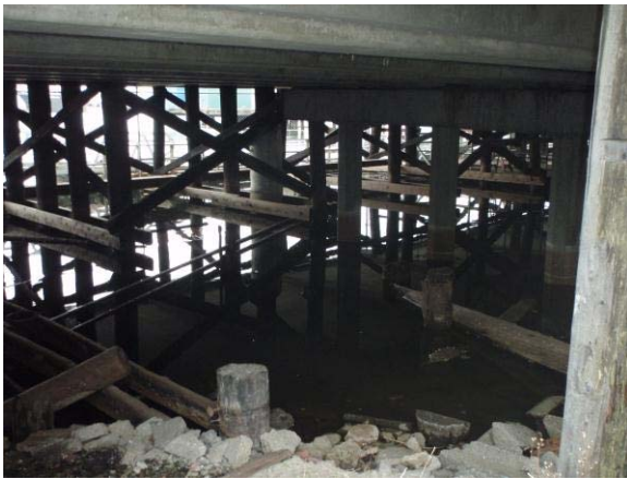
Photo 5. View to the north showing the timber piling supports for the West Bridge; a concrete support for the East Bridge is visible in the foreground. 2011
