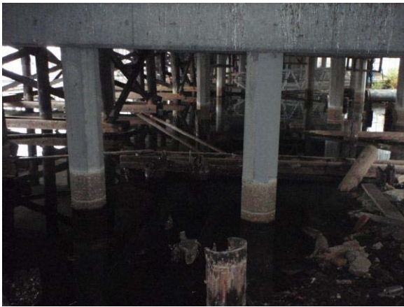
Photo 5. The concrete supports from the 1963 bridge and sawed timber piles from the previous (c. 1917) bridge. View to the north under the East Bridge.
