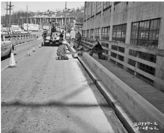
Photo 7. The wooden handrail and traffic curb date to the earlier (c.1917) bridge at this location. This handrail was replaced in 1963 except at the approaches. The traffic curb was replaced in 1988 (Seattle Municipal Archives Photograph No. 70915).
