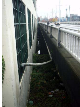
Photo 2. Note the reflection on the water below and pipes leading from the Steam Plant. The sidewalk handrail seen here is from the 1963 design and is based on Standard Bridge Railing Type 3-A.
