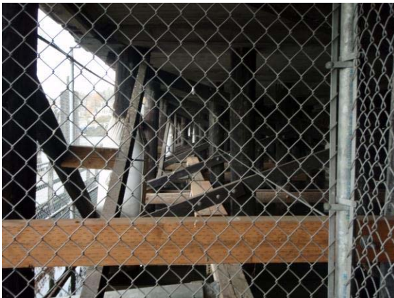
Photo 3. View to the north, showing the cross beams and timber piling supports of the West Bridge. 2011
