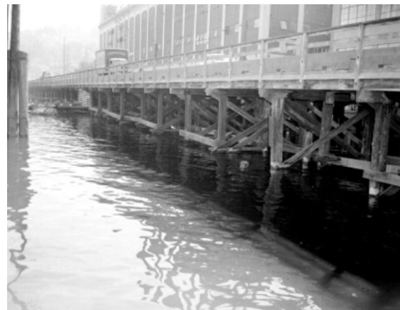
Photo 8. View to the north; note original wooden guardrail and timber supports (Seattle Municipal Archives Photograph No. 41304). 1948
