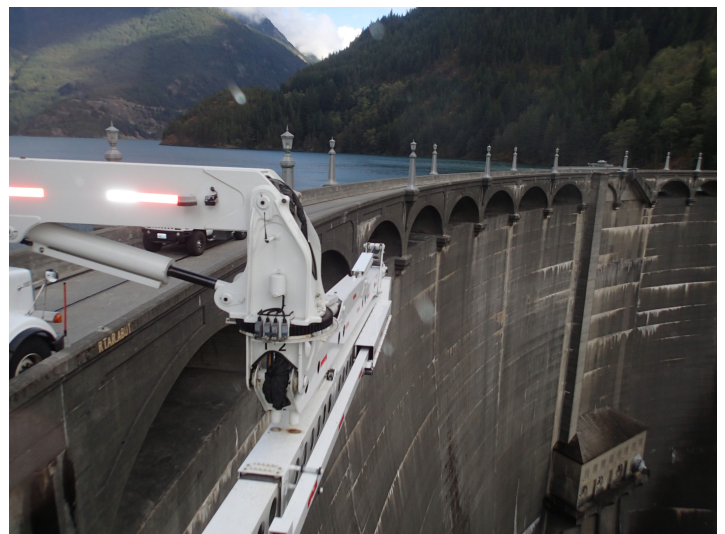
BELOW: Seattle City Light Diablo Dam Bridge Inspection
