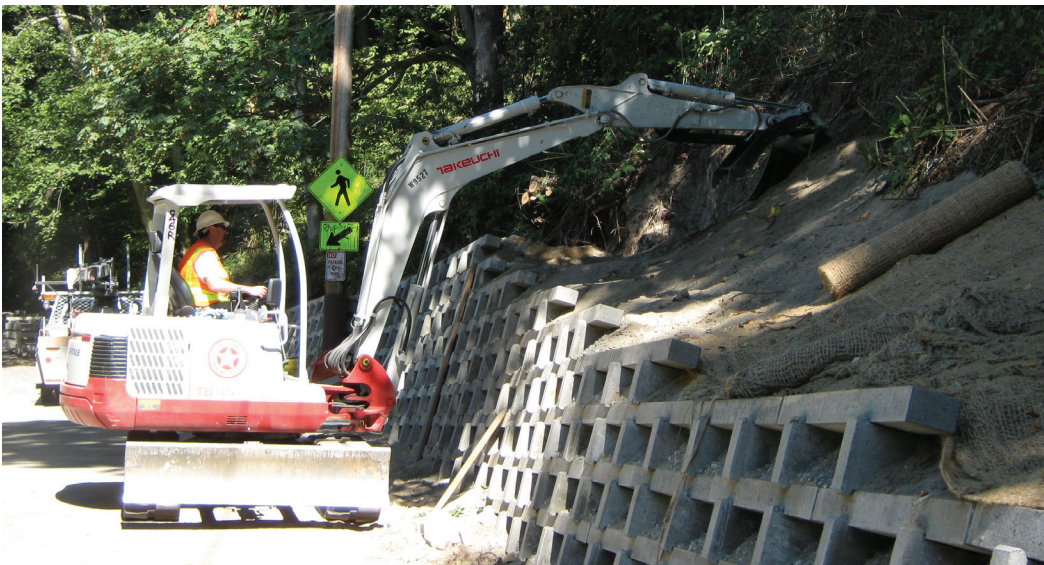
ABOVE: Lakeside Ave S retaining wall between S Judkins and S Norman streets RIGHT: Retaining wall construction
