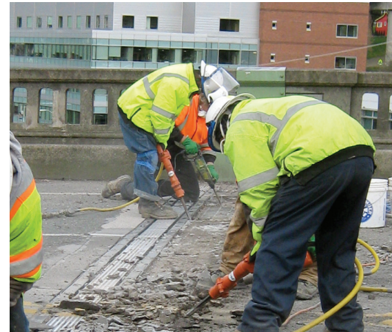
University Bridge expansion joint work
