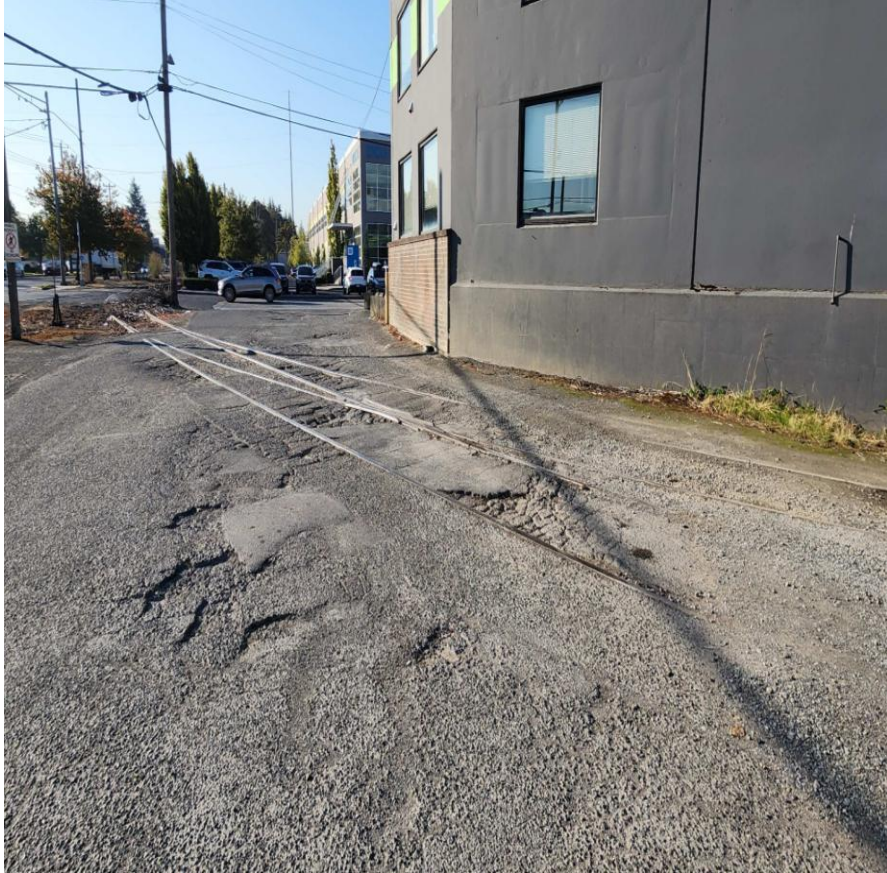
Future rail removal at S Idaho St
