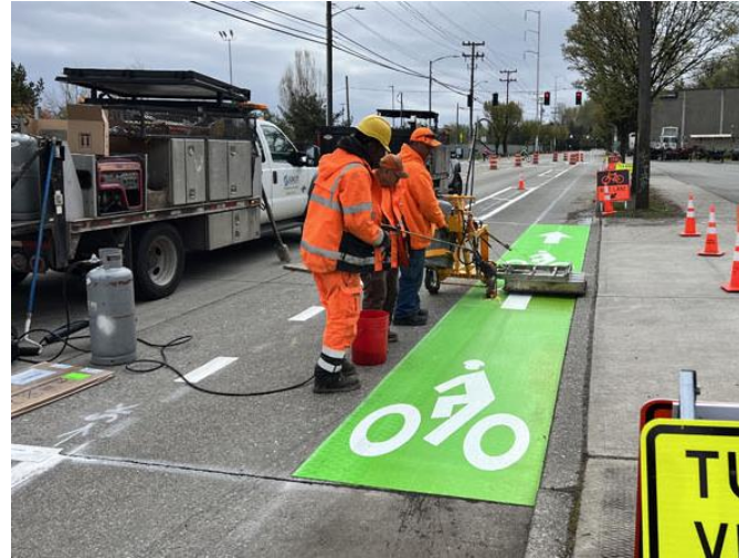
Thermoplastic installation along West Marginal Way SW PBL
