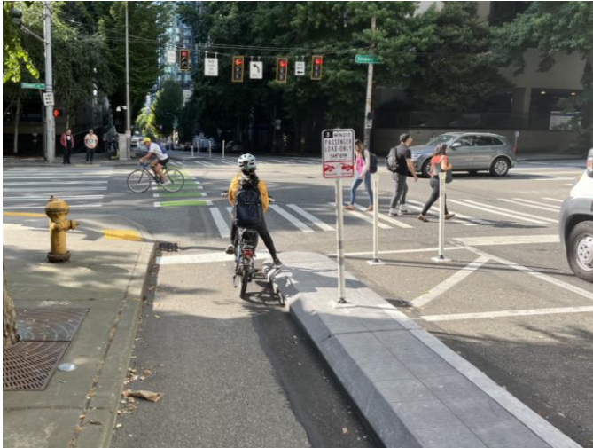
Upgraded curb protection on 8 th Ave PBL
