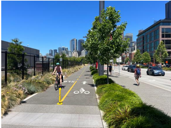
Completed waterfront bike path on Alaskan Way from S King St to Yesler Way
