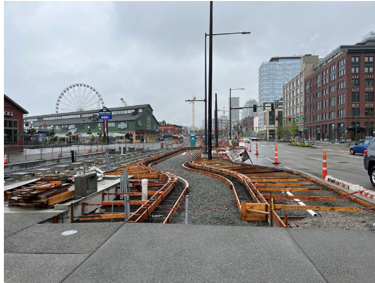
Waterfront bike path under construction between Yesler Way and Virginia St, planned opening by 2024
