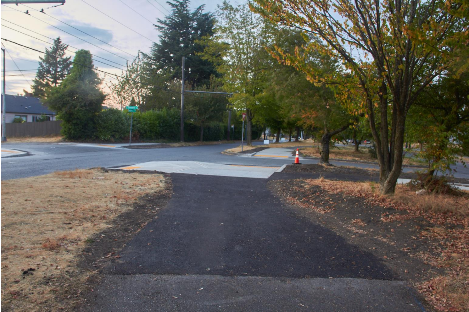
Beacon Ave S path
