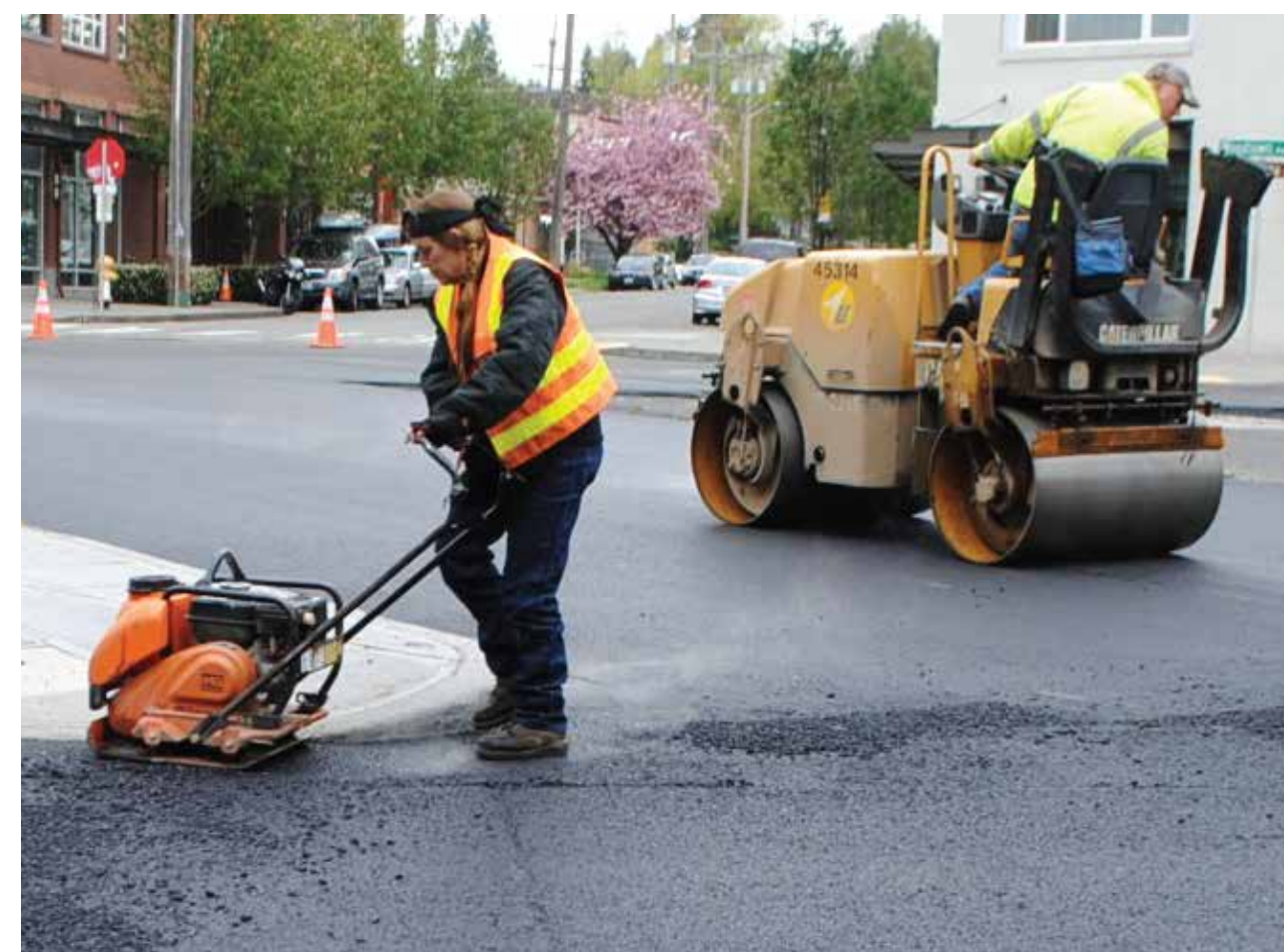
Pavement repair
