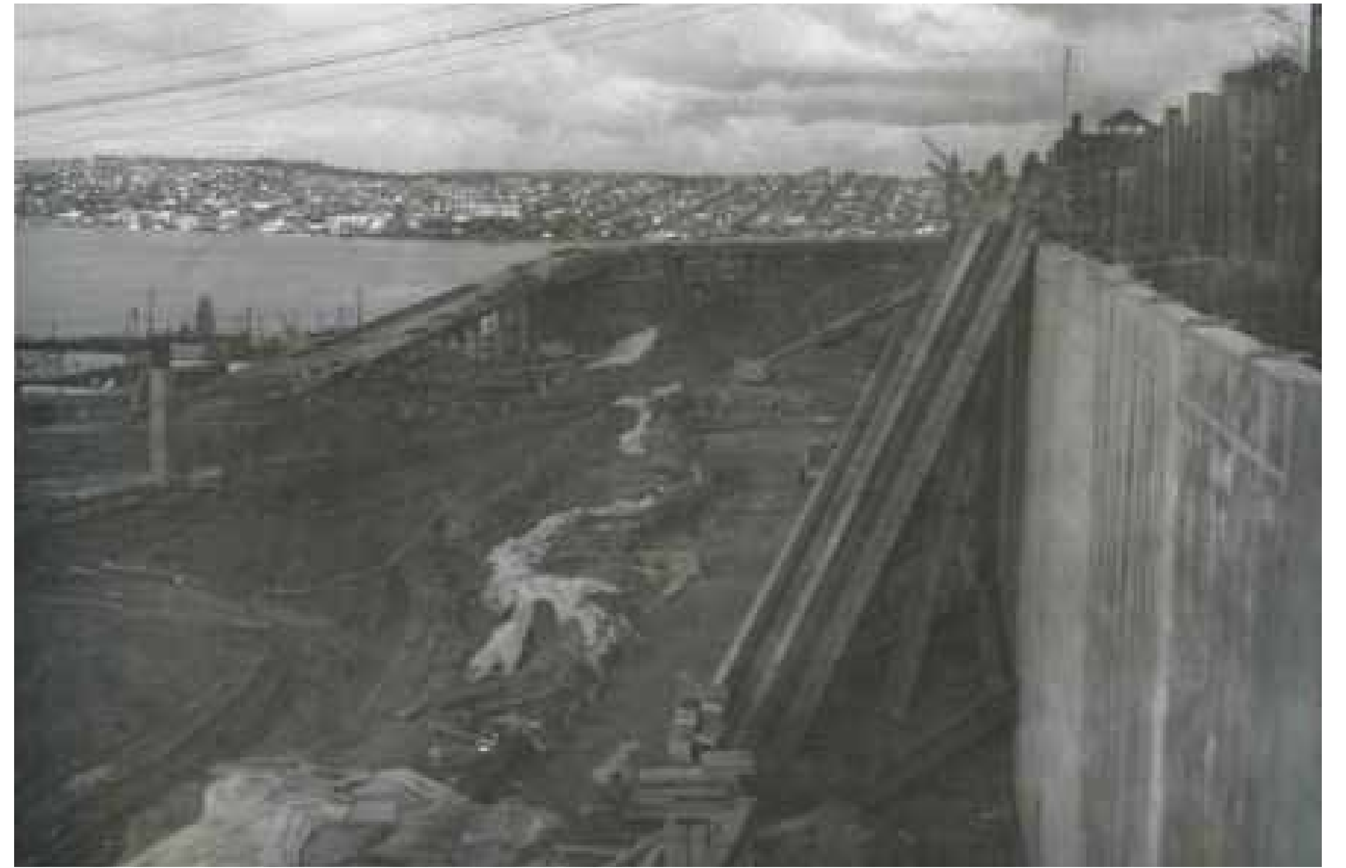
Interstate 5 construction cuts off Melrose Ave and Capitol Hill from Eastlake. Photograph taken by Werner Lenggenhager on November 22, 2012. © Seattle Public Library
