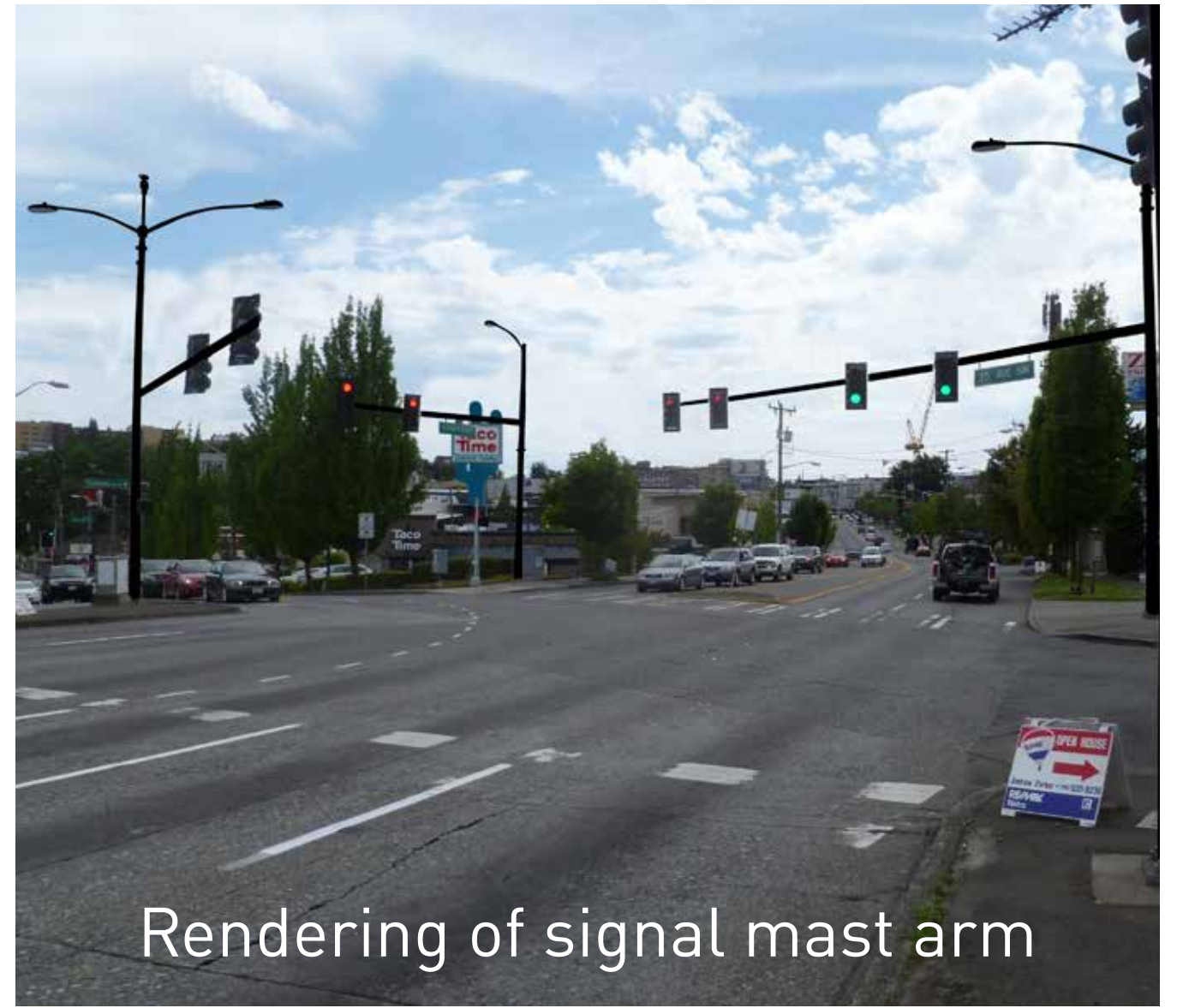
Reduced overhead wires by adding signal mast arms and consolidating utility wires
