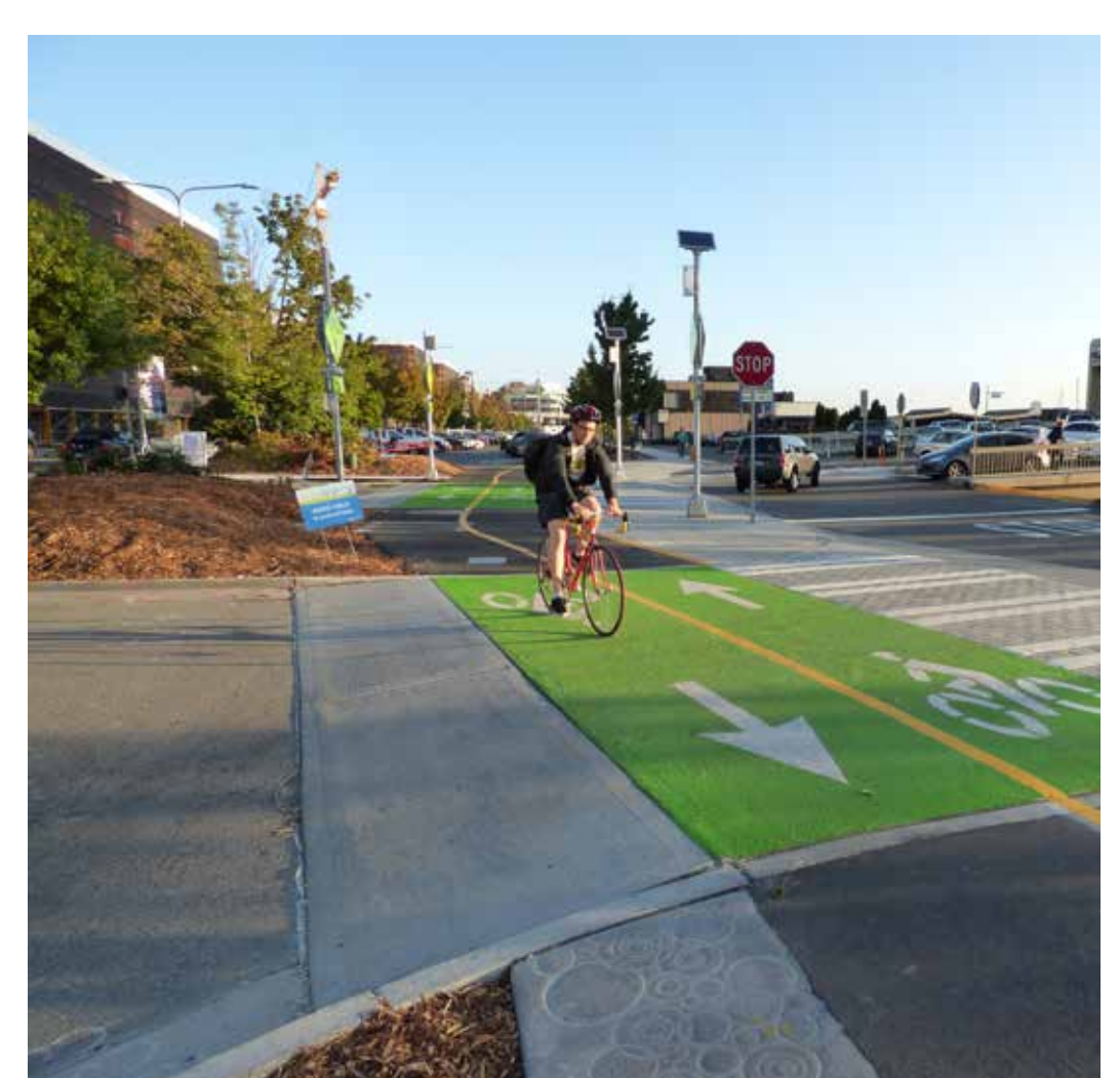
Green paint where PBL crosses driveways
