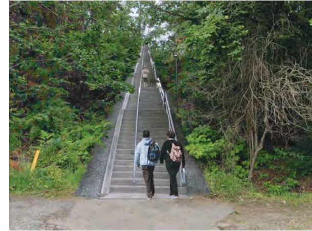
S Henderson Stairway Project https://www.seattle.gov/transportation/SHendersonStairway
