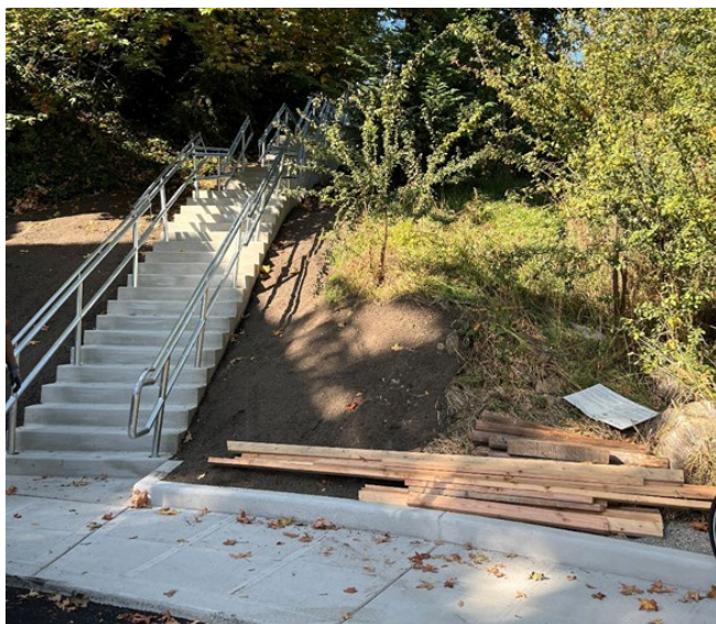
Repaired stairway on S Brandon St.
