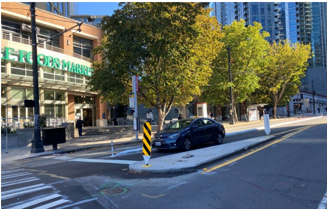
New posts to restrict northbound right turns from Westlake to Denny Way and prevent cars from using the bus-only lane.
