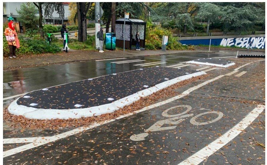
Along NE Campus Parkway, a new type of bike lane barrier made of upcycled tires. Nearby, there is a new asphalt median to separate riders from traffic.
