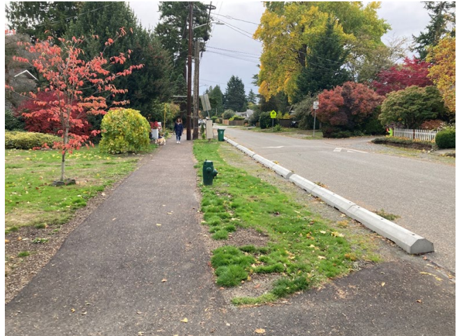
New walkway on Corliss Ave N between N 117th and N 120th streets near James Baldwin Elementary School.
