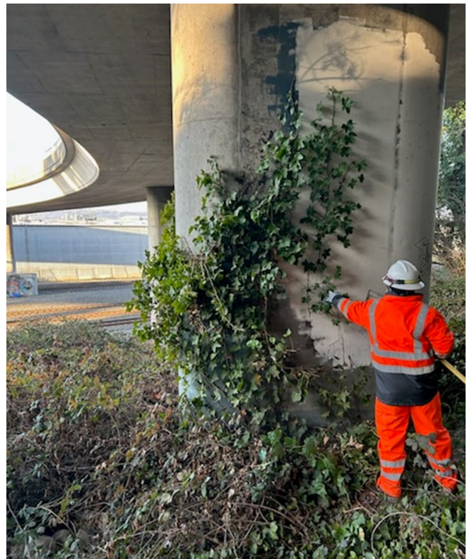
Bridge cleaning on a bridge on S Lucile St.
