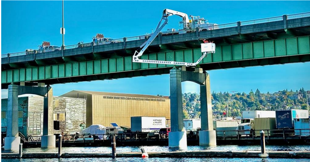
Repairs on Ballard Bridge.
