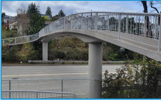
SW Andover St Pedestrian and Bicycle Bridge.
