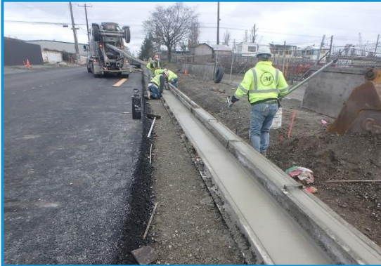
Work on a gutter and curb on S Monroe St.
