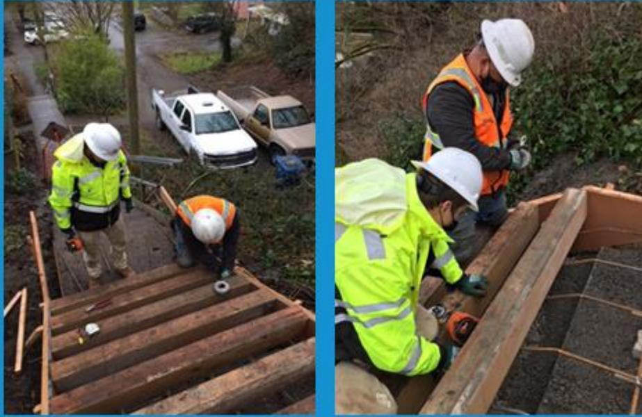
SDOT staff rebuilt the stairway at 10th Ave S & S Donovan St in Q2. To keep our stairways safe and accessible, SDOT inspects the condition of each public stairway across the city and identifies repairs. Repairs range from replacing the handrails to replacing the stairway altogether.
