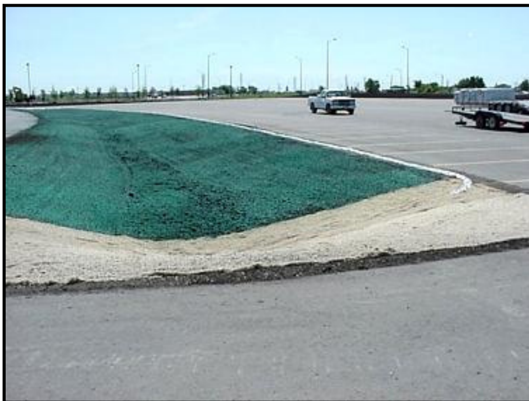
Figure 1. Hydroseeding Method.
