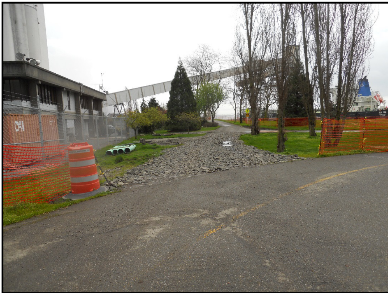
Figure 7. Stabilized Construction Access.
