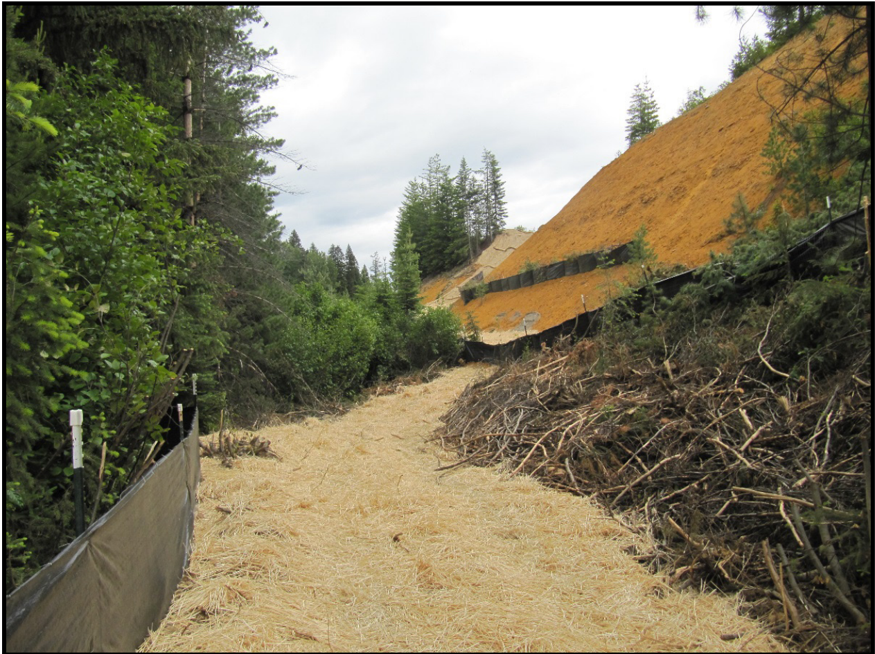
Figure 13. Filter Fence Installed on a Slope.
