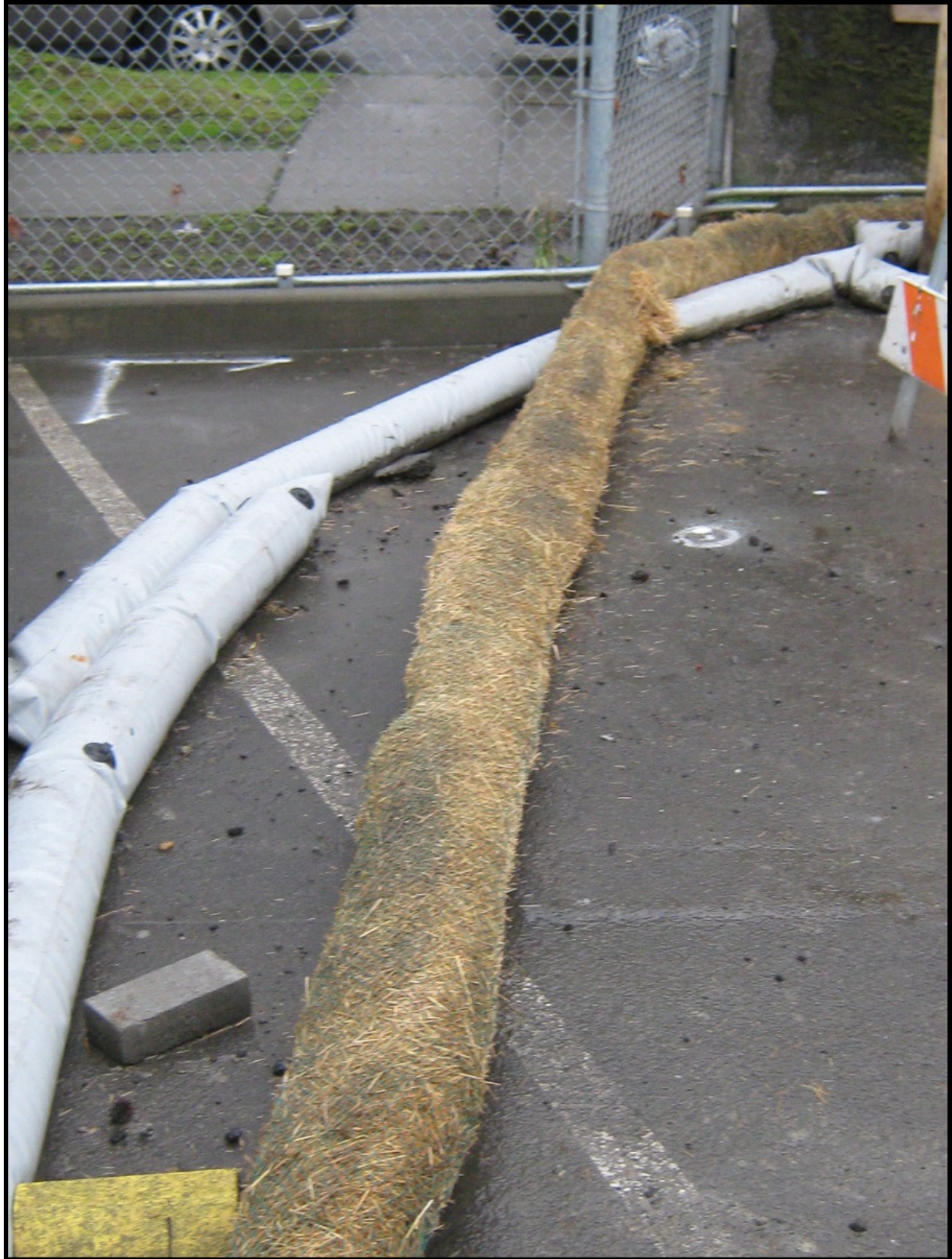
Figure 16. Curb and Gutter Barrier.
