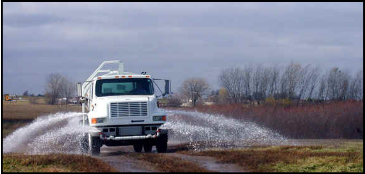
Figure 11. Using a Water Truck for Dust Control.
