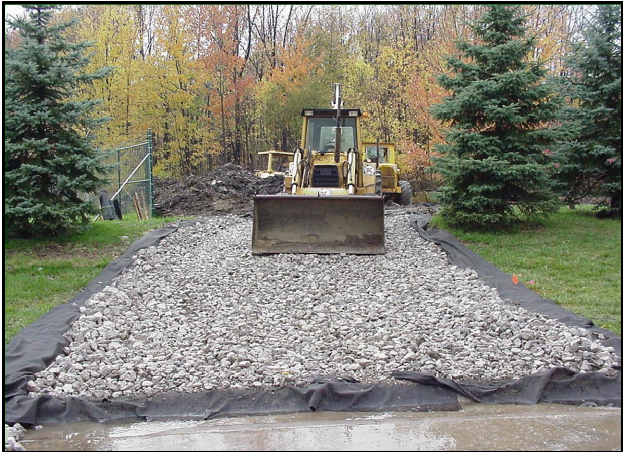
Figure 6. Stabilized Construction Access.
