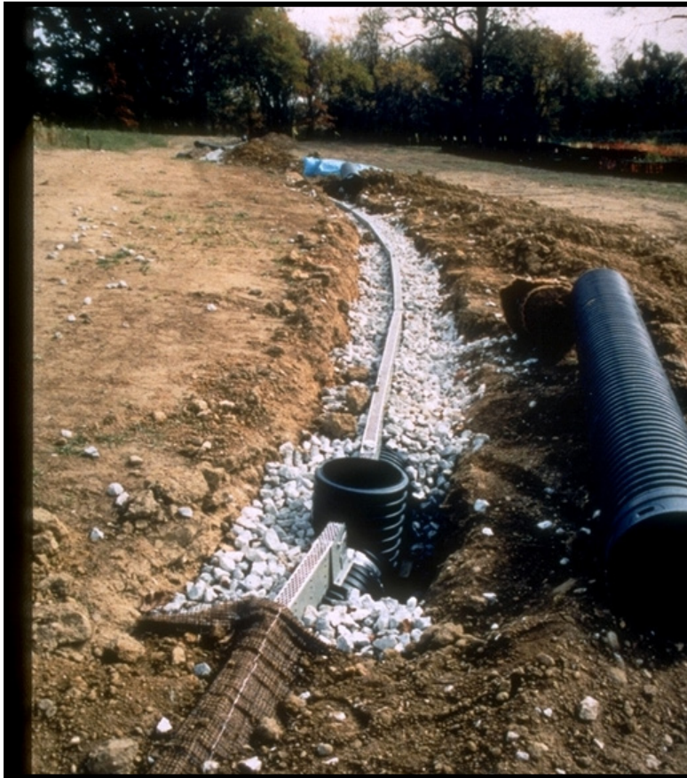
Figure E.7. Level Spreader Prior to Backfill and Downstream Stabilization.
