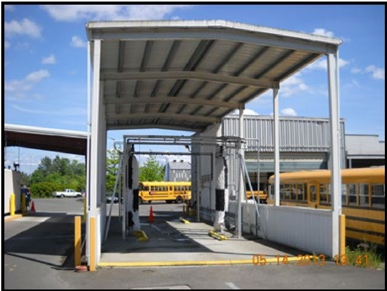
Figure 86. Car Wash Building with Drain to the Sanitary Sewer.
