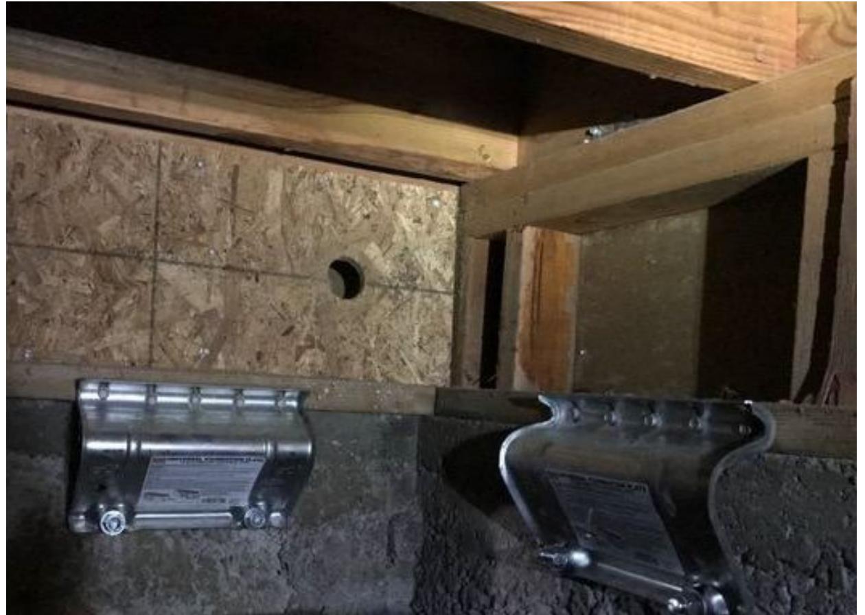
OSB braced wall panel (with hole) and URFP courtesy of Simpson Strong Tie
